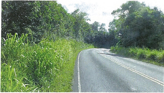
Property on left, Kūhiō Highway going towards Hanalei
