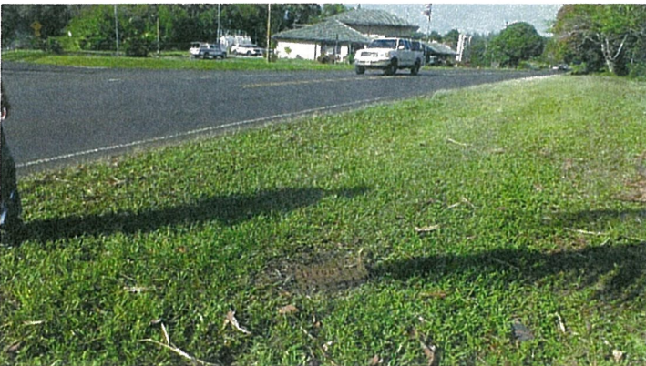
Kūhiō Highway at Hanalei Plantation Road. Note Hawaiian Tel underground utility and 5000-gal AST on adjacent site.
