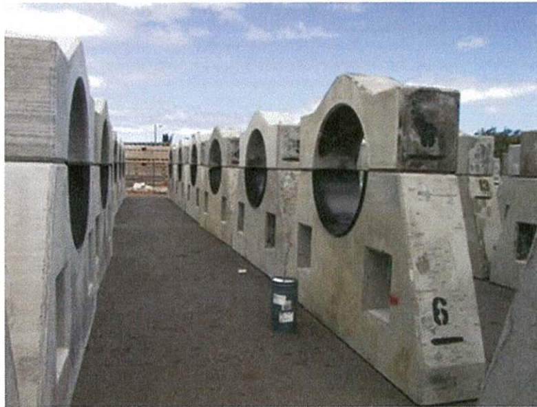
Photo 2. Example of gravity concrete anchors or "collars" for an HDPE Pipe at Keahole Pt., Hawaii. Source: Makai Ocean Engineering, Inc. ( https://www.makai.com/ )
