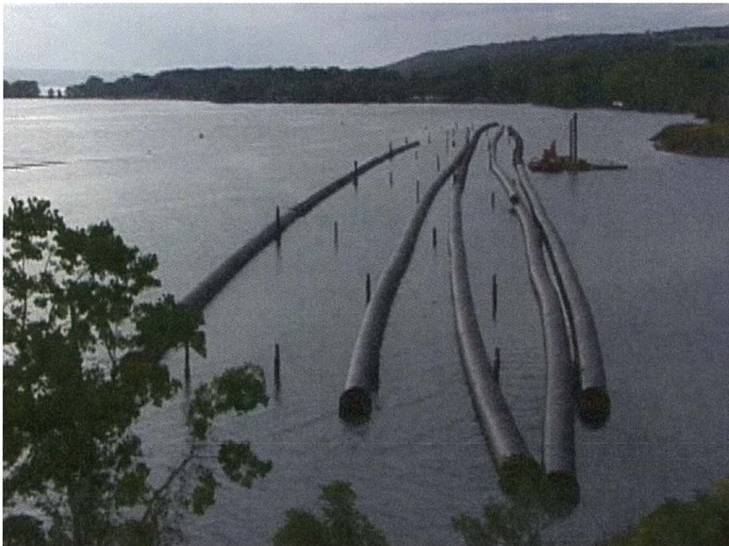
Photo 1. Example of Stored Floating Pipeline with Stiffeners and Anchor Weights Being Attached. Source: Makai Ocean Engineering, Inc. (FEIS, HSWAC) (Cardno TEC, Inc., 2014)
