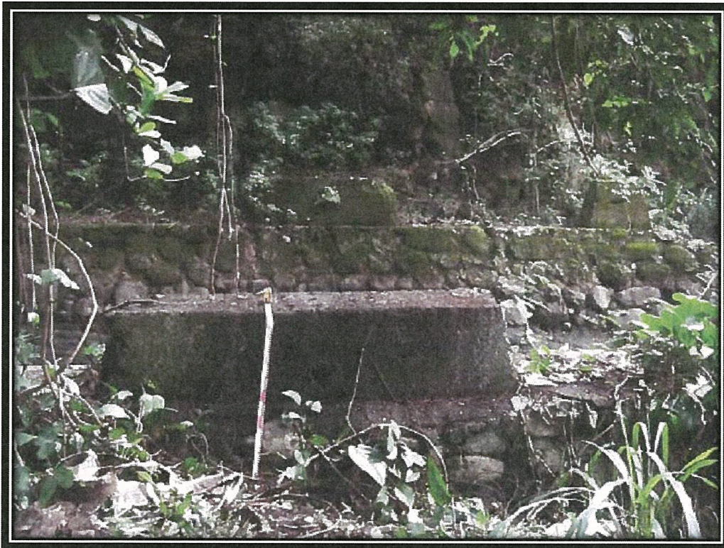
Photo #2 Trestle Foundation
