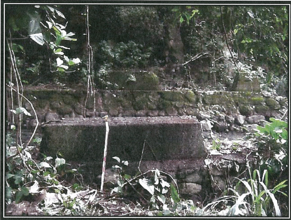
Photo #2 Trestle Foundation
