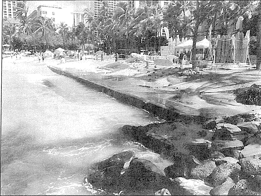
EXHIBIT 6: Exposed Waikiki Tavern concrete foundation (August 21, 2017 photo)
