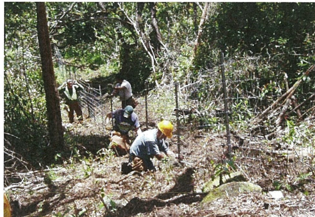
Ungulate fencing installation
