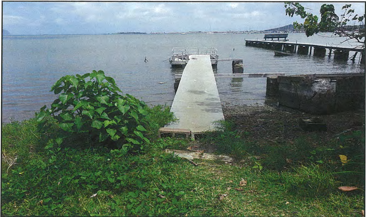
Photo looking north towards the pier.
