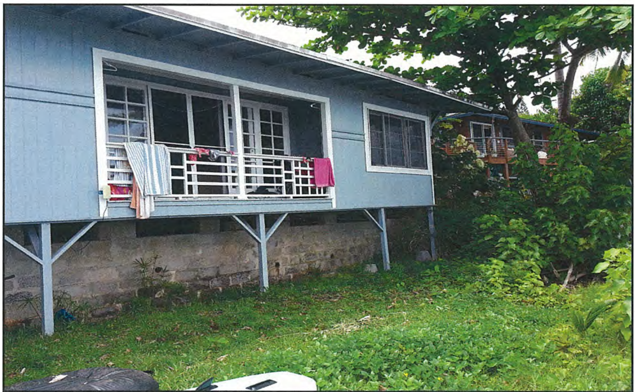
Photo looking southwest towards the house encroachment.
