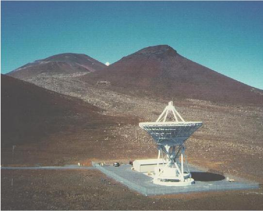
The Mauna Kea Very Long Baseline Array (VLBA) is one unit in an integrated system of ten identical radio telescopes stretching from the U.S. Virgin Islands to Hawai'i, which are operated remotely from Socorro, New Mexico. Each VLBA station consists of a 25m antenna and an adjacent control building. The ten stations work together as one single instrument. It is in the lower summit region at approximately 3700 meters elevation.
