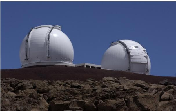
The twin Keck Observatory telescopes primary mirrors are 10-meters, each composed of 36 hexagonal segments that work in concert as a single piece of reflective glass.
