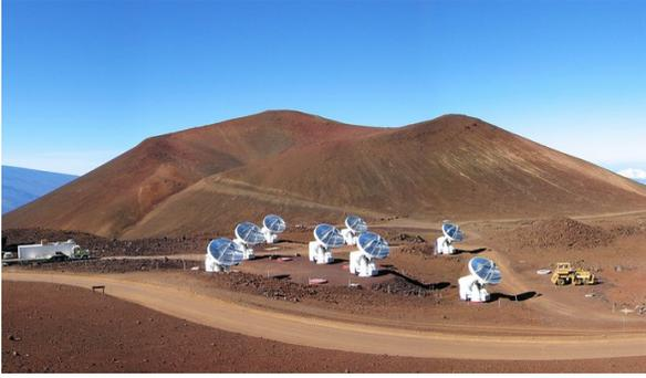
**SMA** consists of eight 6-meter radio telescopes that operate as one unit. The telescopes can be arranged in varying configurations using 24 concrete pads. SMA is located at the base of Pu'u Poli'ahu in an area informally known as "Submillimeter Valley."
