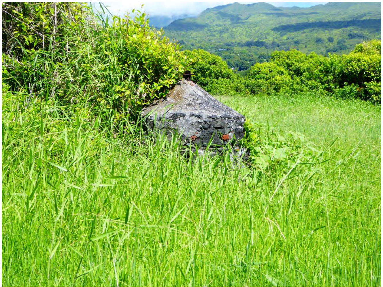
Carin anchor for sugar mill chimney
