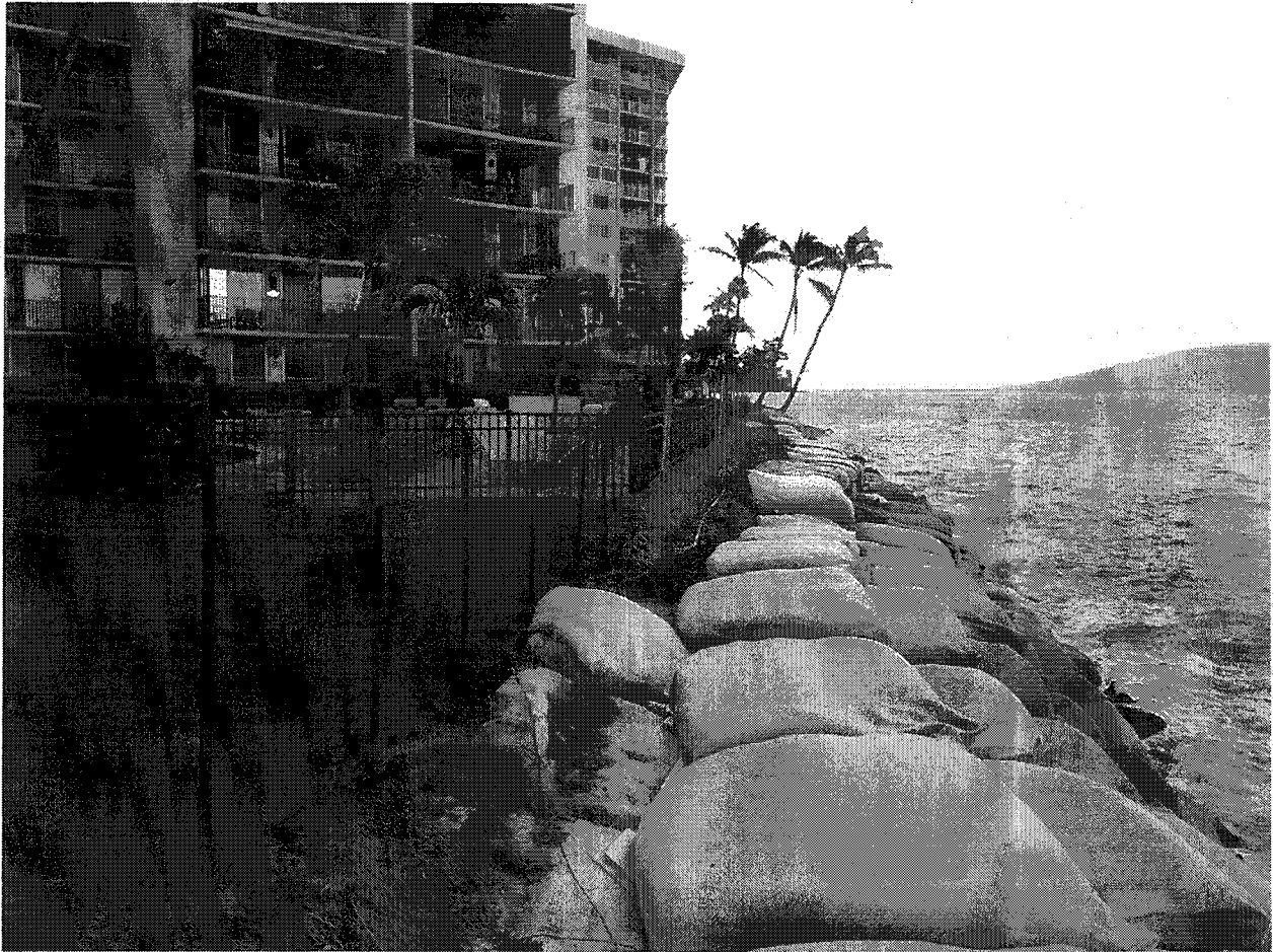
Looking southwest – sandbags adjacent to the pool area. Between north and south building.
