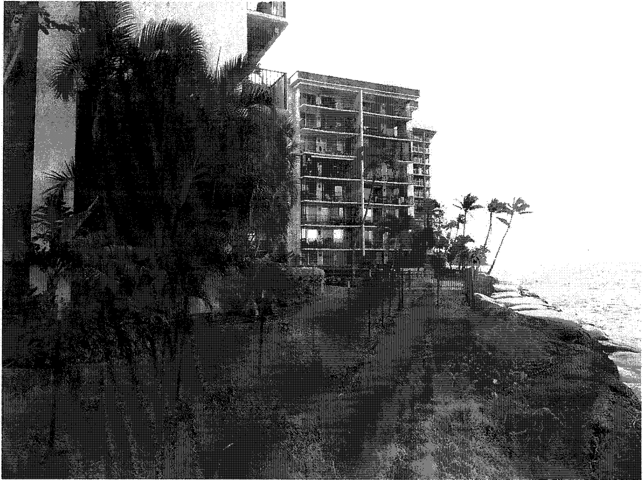
Looking southwest – north building area.
