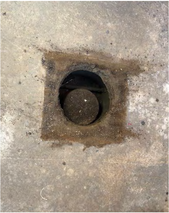
Photo 22: Hot Spots – view of access port in concrete pavement reportedly for a septic tank.
