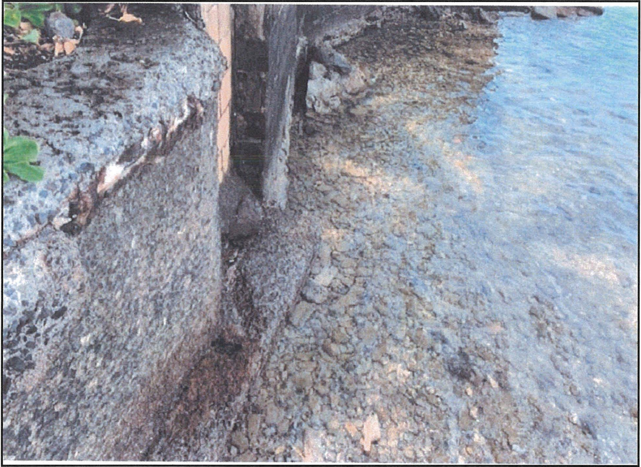
Photo looking at the south corner of the seawall. Photo showing additional concrete footing.
