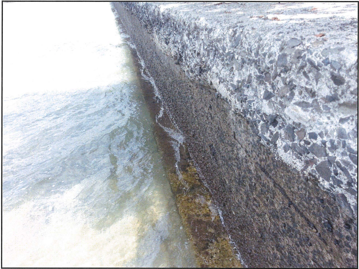
Photo looking north showing footing encroachment extending beyond the seawall face. Note the seawall overhang at the top of the seawall.
