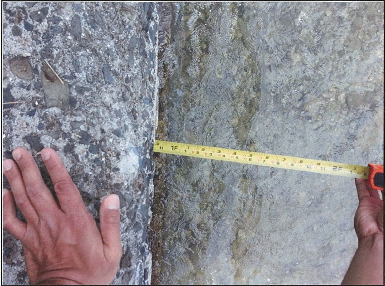
Photo showing depth of seawall overhang. Note that the seawall footing can be seen at the water line.
