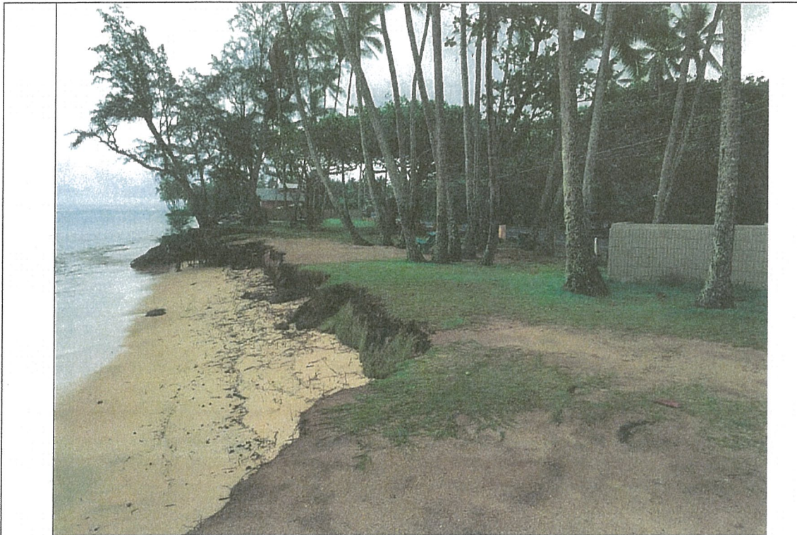
Figure 2: Shoreline erosion at Punalu'u Beach Park with Kamehameha Highway in the background.
