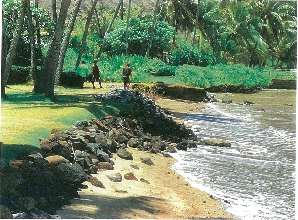
Figure 4 - Rocks Actively Being Placed Along Scarp Located Seaward of Residential Parcel and Located on and Seaward of Subject Beach Reserve Parcel, Facing Southeast
