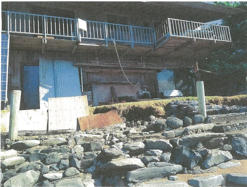
Figure 4 – Subject Seawall, Facing Mauka
