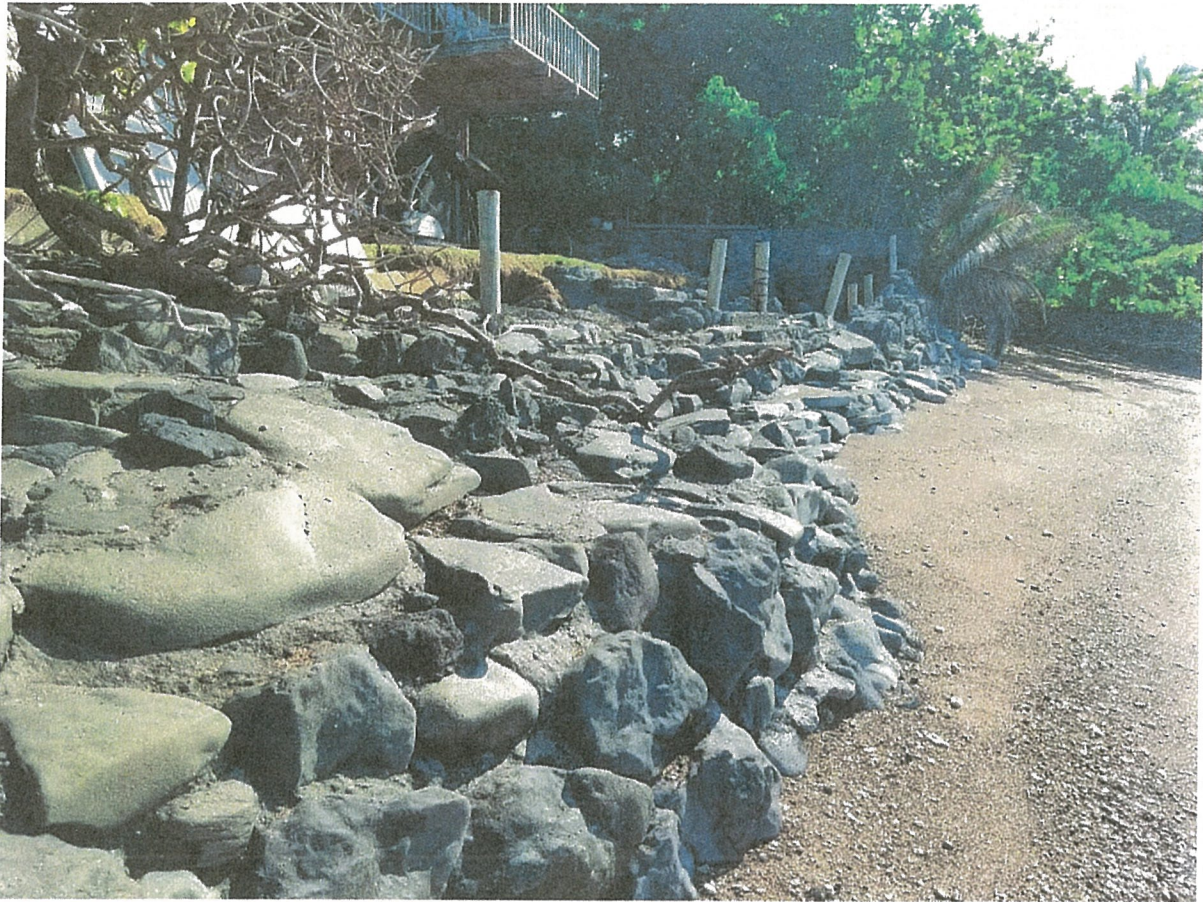
Figure 5 – Subject Seawall, Facing East
