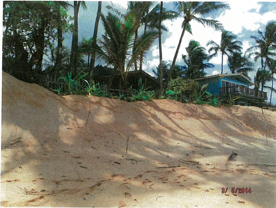
Figure 9 – March 5, 2014 Photo Showing Wall's Existing Condition Following Sand Push
