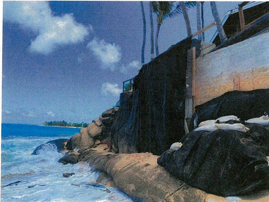
Figure 14 – August 15, 2020 Photo Showing Alleged Construction
