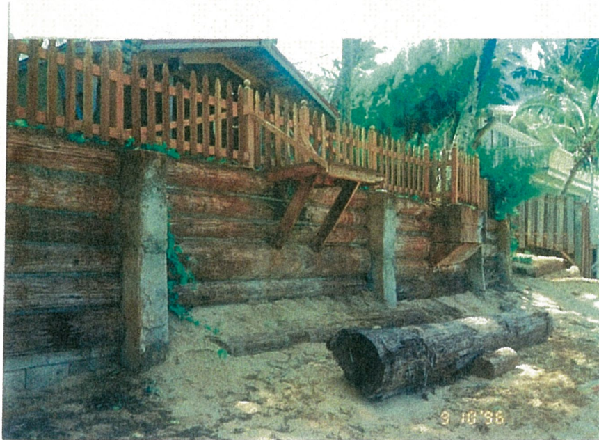
Figure 5 – September 10, 1996 Photo Showing Wall's Existing Condition
