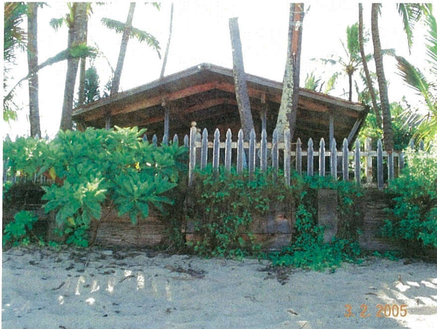
Figure 7 – March 2, 2005 Photo Showing Wall's Existing Condition
