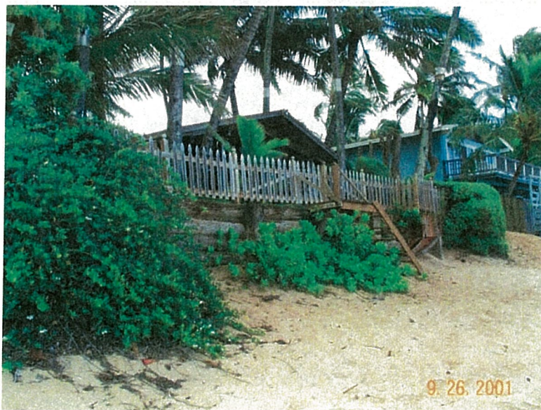
Figure 6 – September 26, 2001 Photo Showing Wall's Existing Condition
