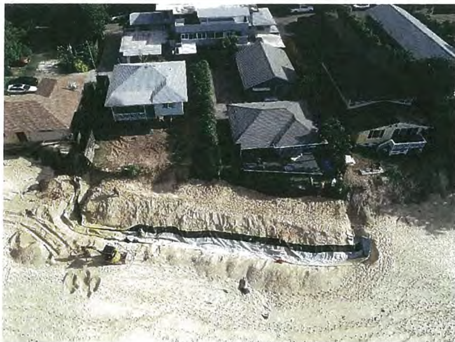
Figure 18: December 10, 2020 OCCL Site Visit Photo Showing Unauthorized Work and Installation of Large Sand-Filled Burrito
