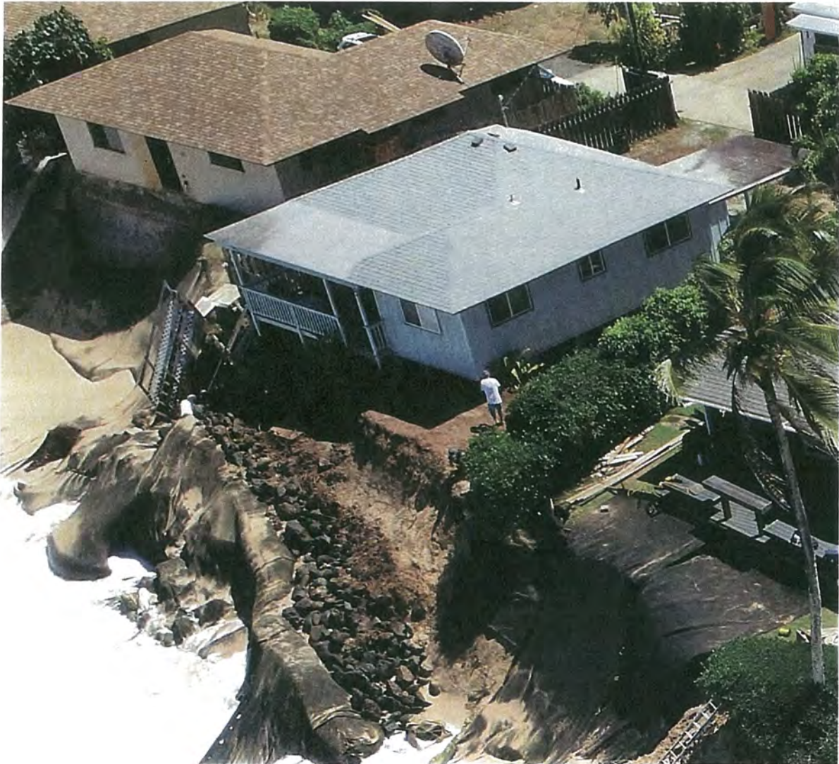
Figure 13: September 30, 2020 OCCL Site Visit Photo Showing Unauthorized Work & Makeshift Rock Revetment
