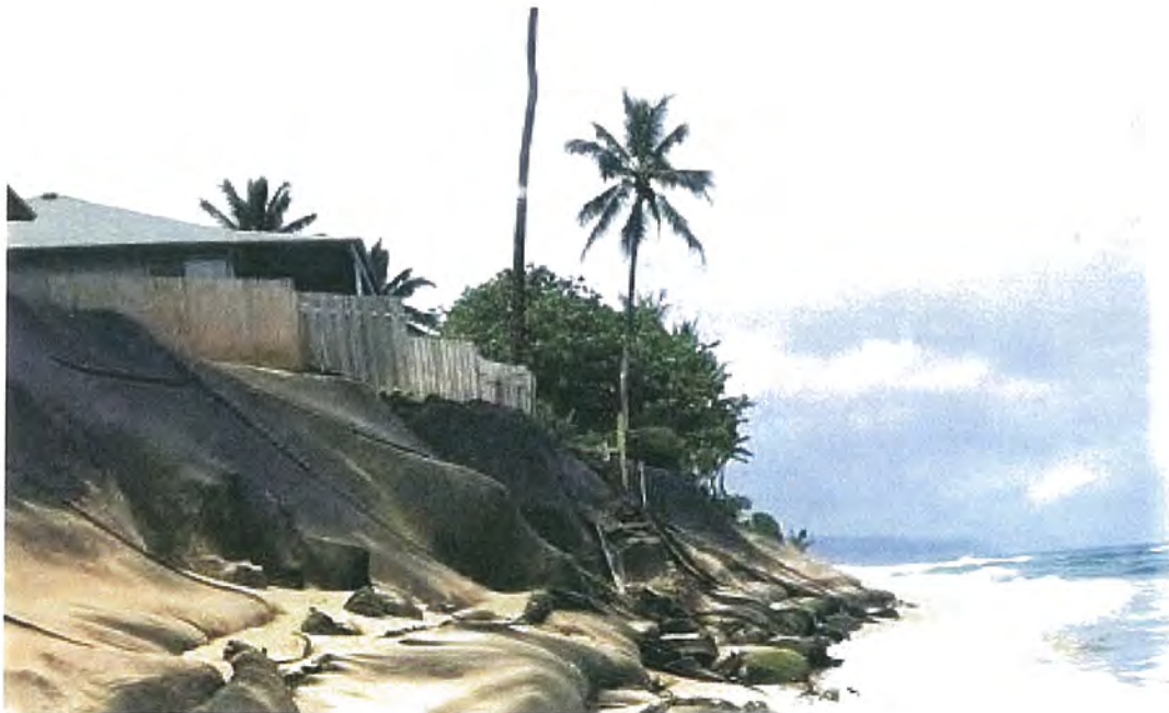
Figure 8: September 17, 2018 Photo Showing Subject Property & Temporary Erosion Control
