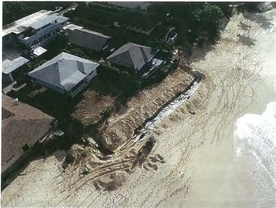
Figure 17: December 10, 2020 OCCL Site Visit Photo Showing Unauthorized Work and Installation of Large Sand-Filled Burrito
