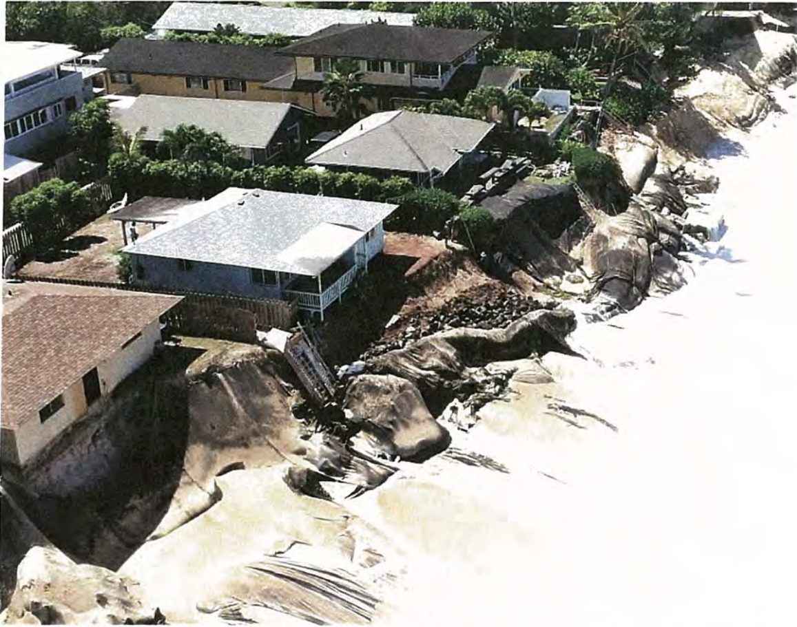
Figure 12: September 30, 2020 OCCL Site Visit Photo Showing Unauthorized Work & Makeshift Rock Revetment
