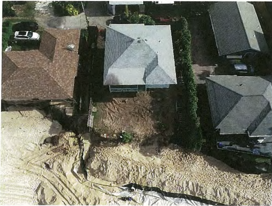
Figure 19: December 10, 2020 OCCL Site Visit Photo Showing Unauthorized Work and Installation of Large Sand-Filled Burrito
