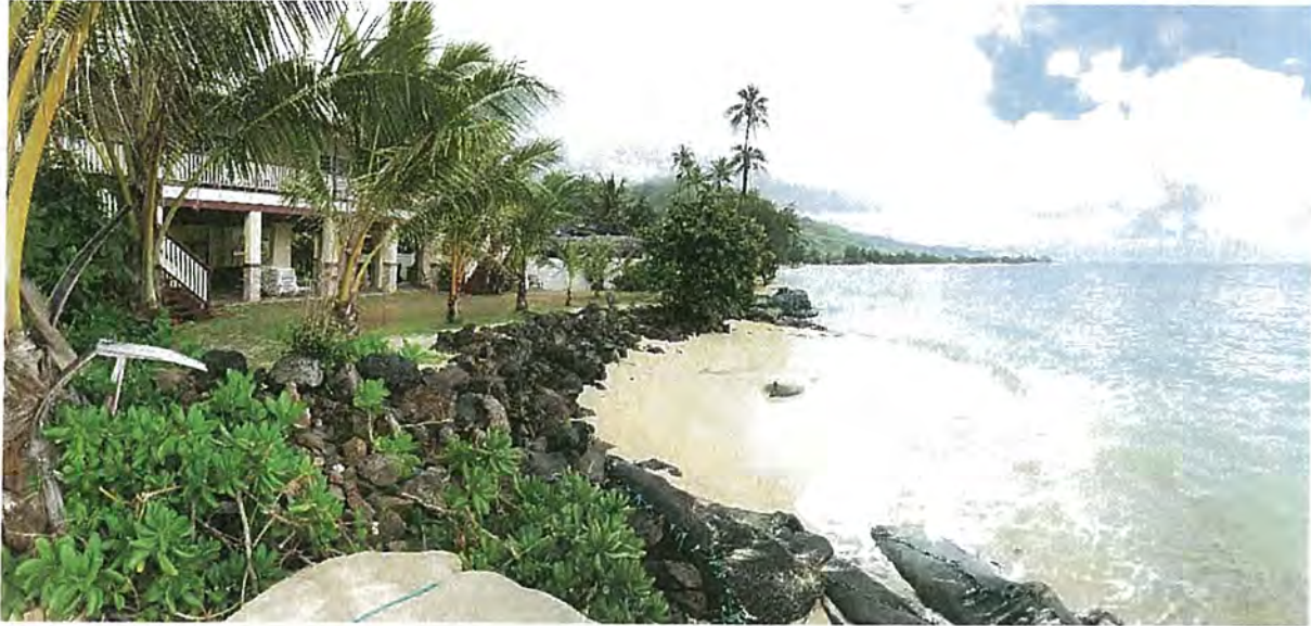
Figure 18: July 2, 2020 OCCL Photo of Alleged Unauthorized Rock Revetment
