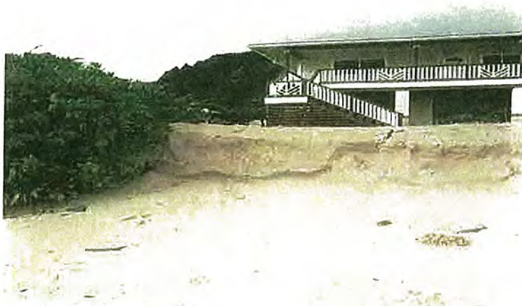
Fields erosion scarp at east side of shoreline July, 2014
