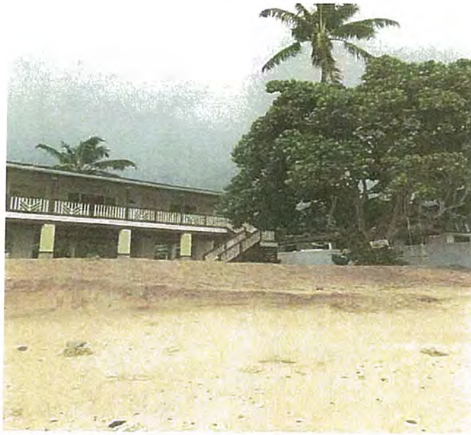
Figure 9: July 2014 Photo Showing Property's New Residence & Erosion Scarp
