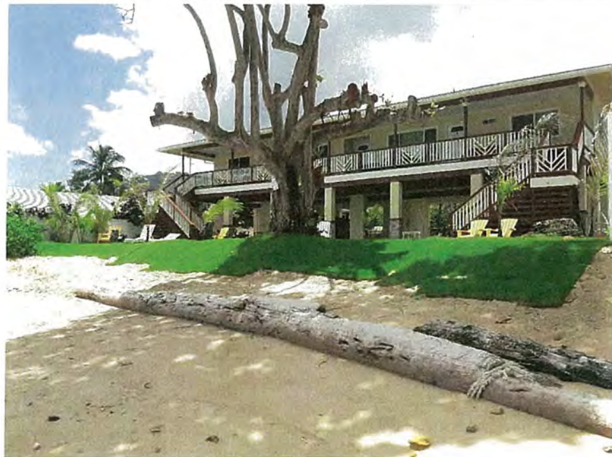
Figure 14: April 18, 2017 OCCL Photo Showing Property's Shoreline
