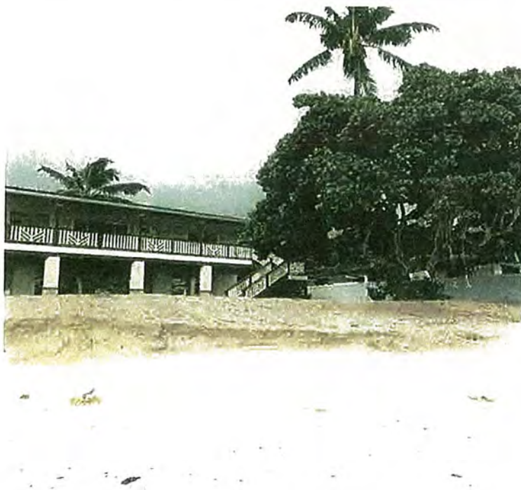
Fields erosion scarp at center of property July, 2014
