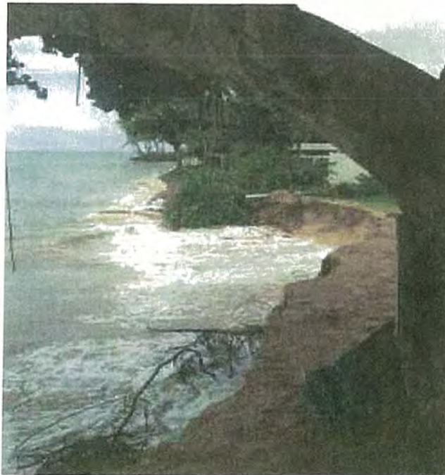
Figure 10: August 8, 2014 Photo Showing Erosion Scarp After Hurricane Iselle
