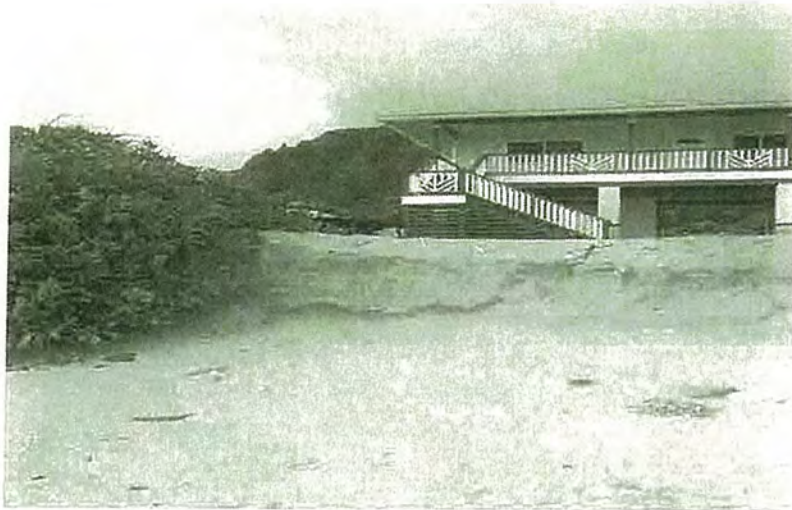
Fields erosion scarp at east side of shoreline July, 2014
