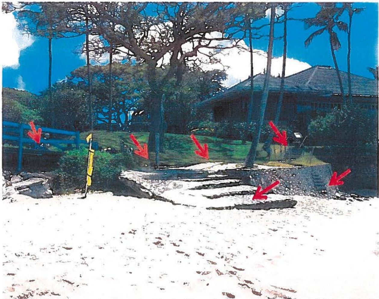
Exhibit 1 - Hardscape to be removed at Kapalua Bay and replanted with native beach / dune friendly vegetation. Two new public beach access paths would be located in the middle of the bay at environmentally appropriate gentler grades with signs.
