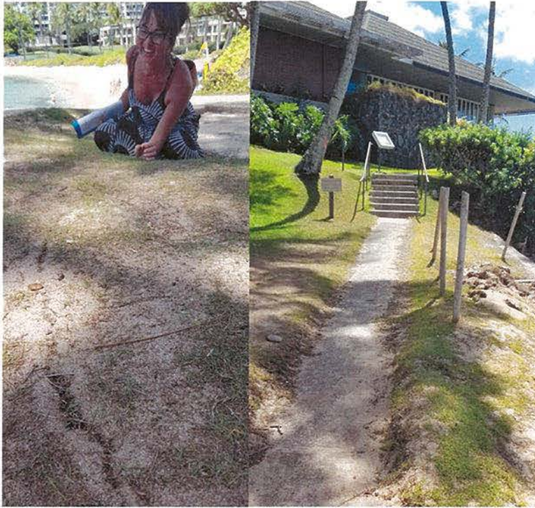
Fissure cracks and a sinking walkway are indicative of the sink hole and its risk of collapse.
