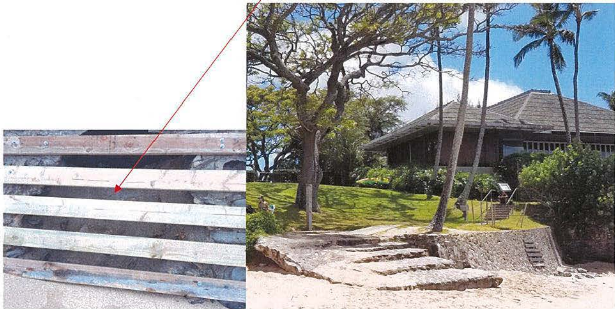
Breach in the wall (top) stabilized in 2016 with wood slats (bottom) and geotextile fabric. (Photos: December 2015, March 2016).
