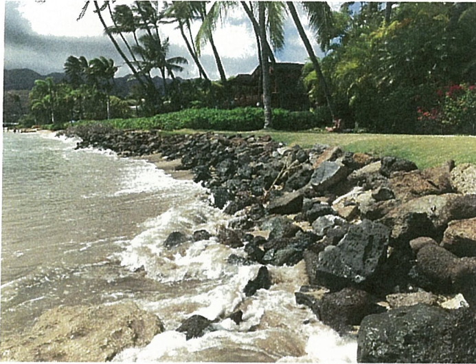
Figure 3 – Rock Revetment Observed by OCCL Staff on July 9, 2020, Seaward of TMK: (1) 3-9-002:003
