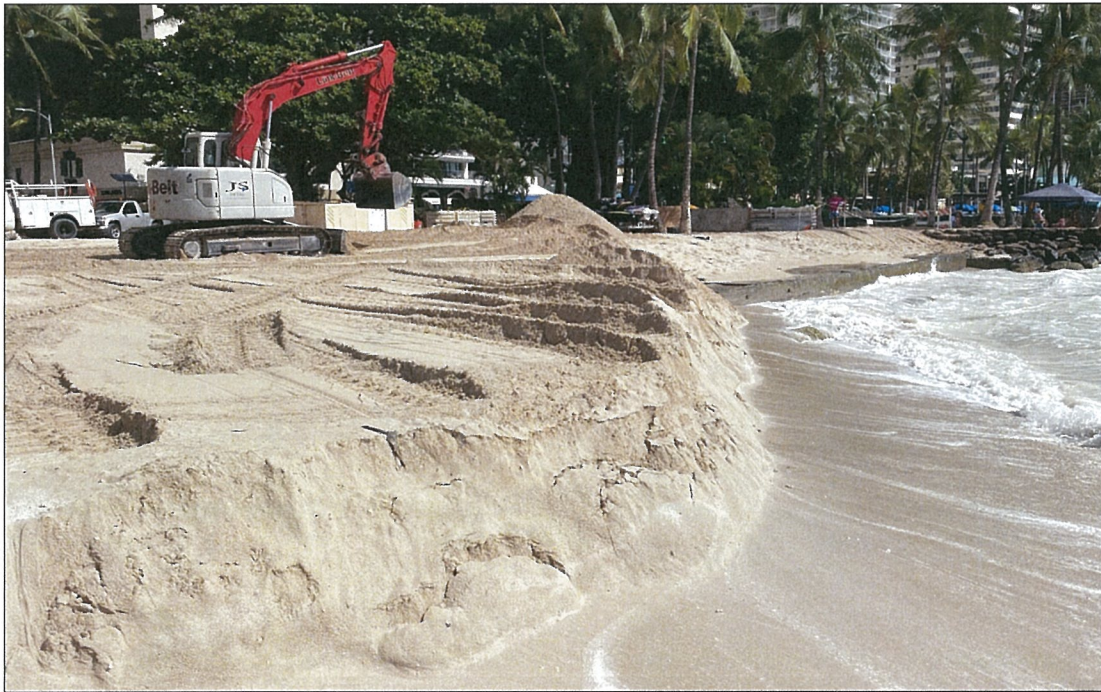
Figure 2. Placement of sand on Kuhio Beach in Waikiki, Oahu, in which sand was sourced from an adjacent area inside the Ewa swim basin.
