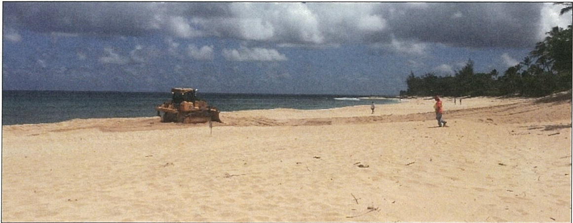
Figure 1. Sand pushing effort undertaken to restore a backshore berm at Pupukea, Oahu
