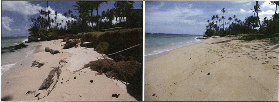
Figure 3. Stabilized beach condition prior to (left) and following (right) completion of Stable Road groin field project on the island of Maui.
