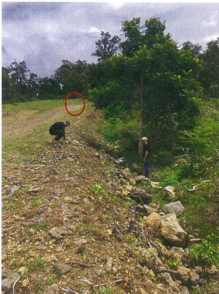
#32 Encroachment of 19.5 ft. Grading over 5 ft tall. Boundary pin in red circle
