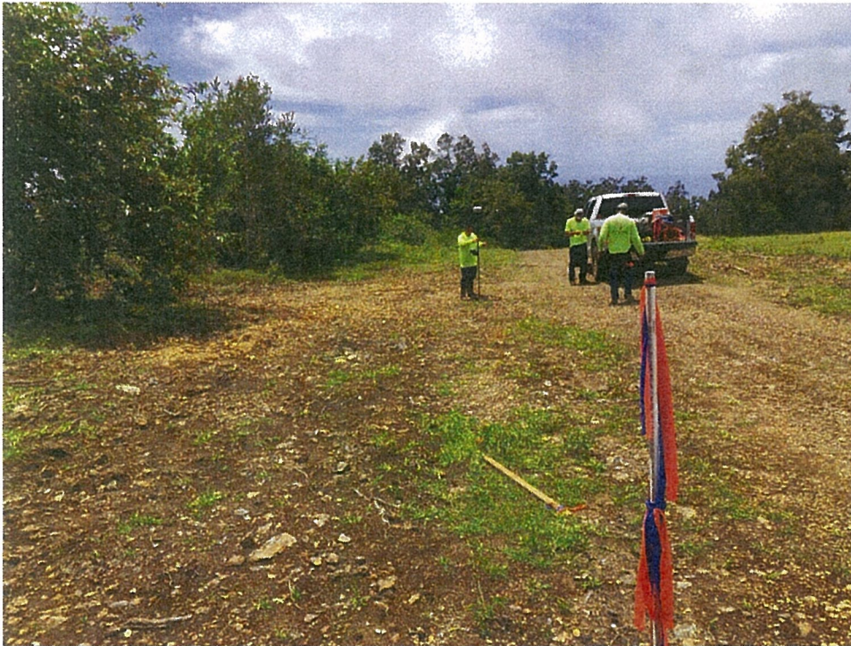
Surveyors marking boundary. Boundary on flagged pole with bulldozing encroachment visible on left
