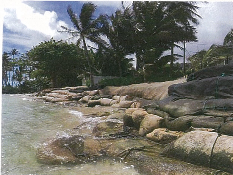
Johnson shoreline protection structure deflating and coming apart 10-26-18
