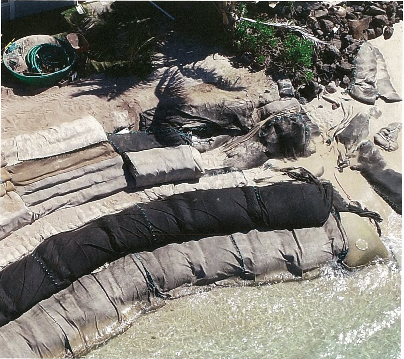
Figure 3: May 29, 2020 OCCL Photo Showing the Installation of Unauthorized Erosion Control Materials
