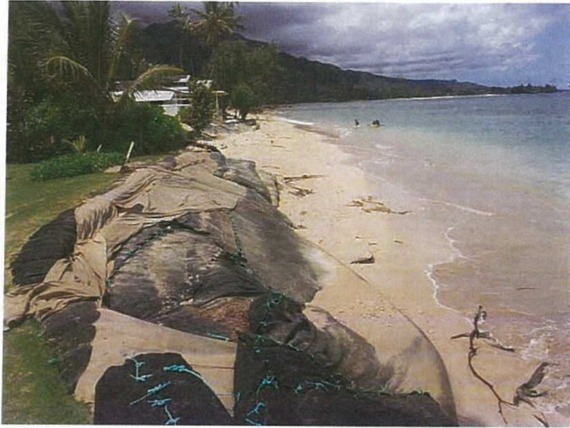
Johnson shoreline structure deflating and coming apart 06-28-19
