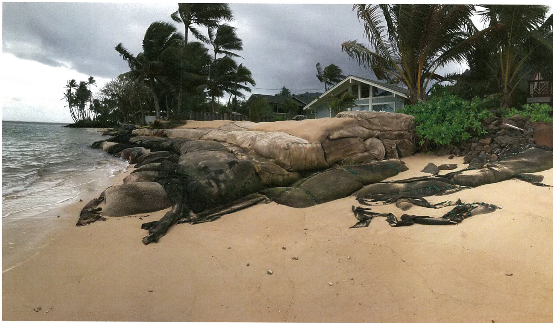
Figure 6: March 17, 2021 OCCL Photo Showing Property's Shoreline Structure Consisting of Several Rows of Unauthorized Erosion Control Materials
