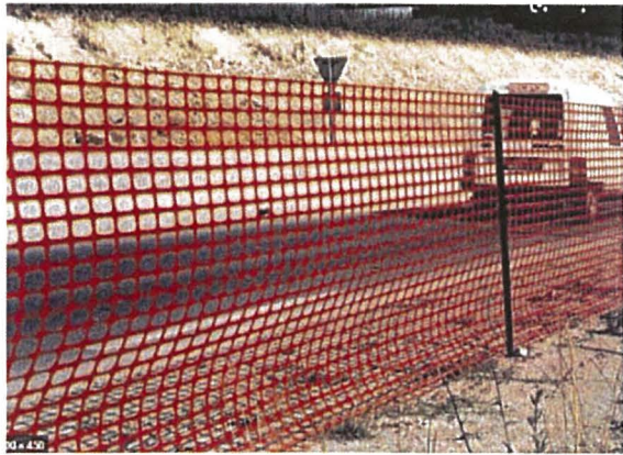
IMAGE: 4' ORANGE DIAMOND NET SAFETY FENCE W/HOG WIRE AND METAL STAKE SUPPORTS
