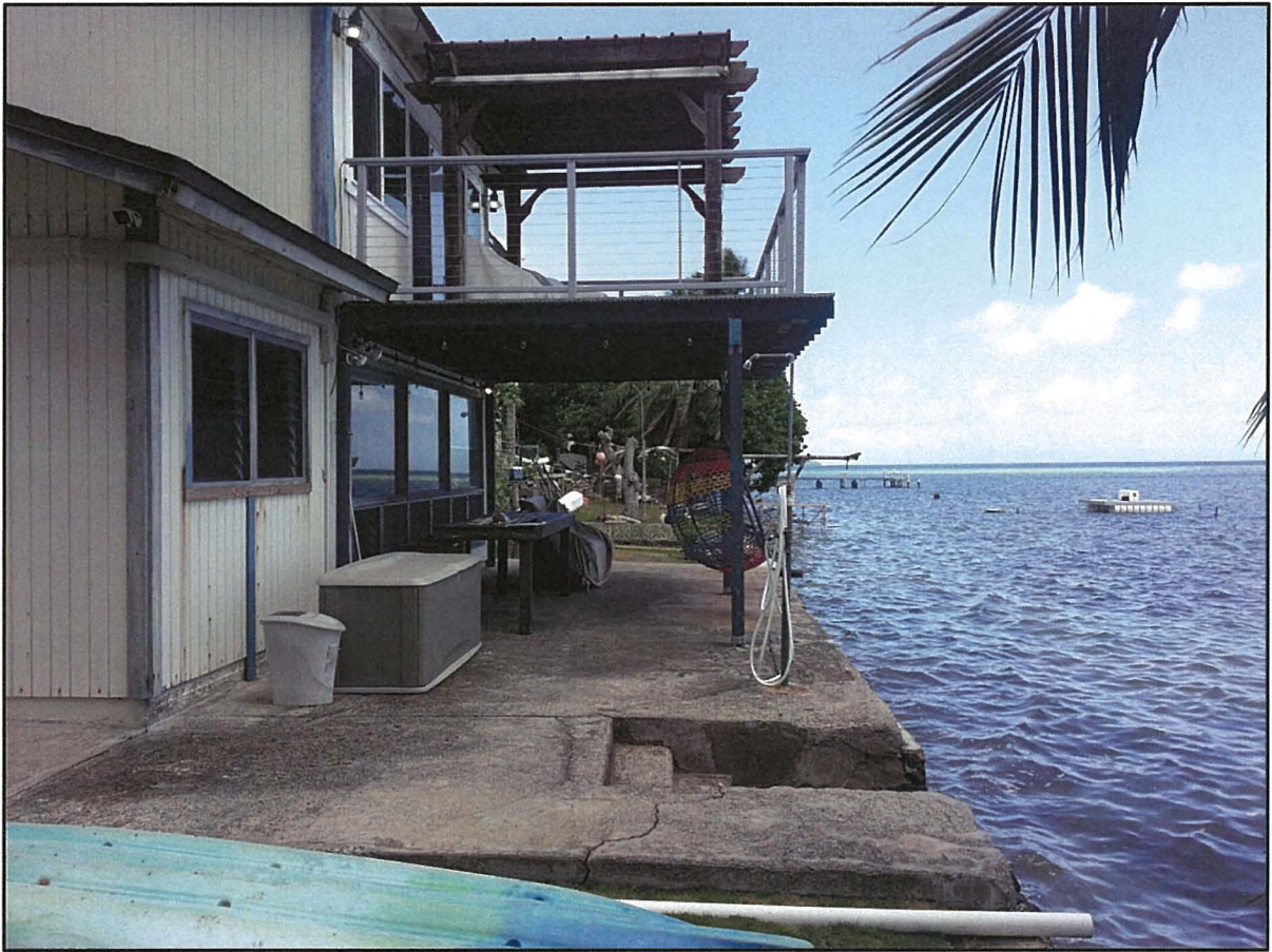
Note: Photo showing reclaimed (filled) land area and no pier. Photo taken facing northwest. Photo taken on August 14, 2019.
