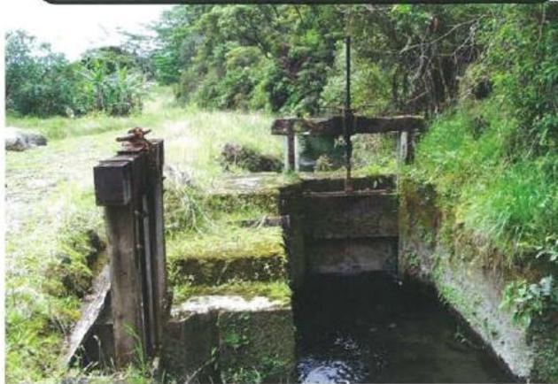
**2017. Gate Valves Removed. No way to regulate flow or prevent damage from storm events.**
