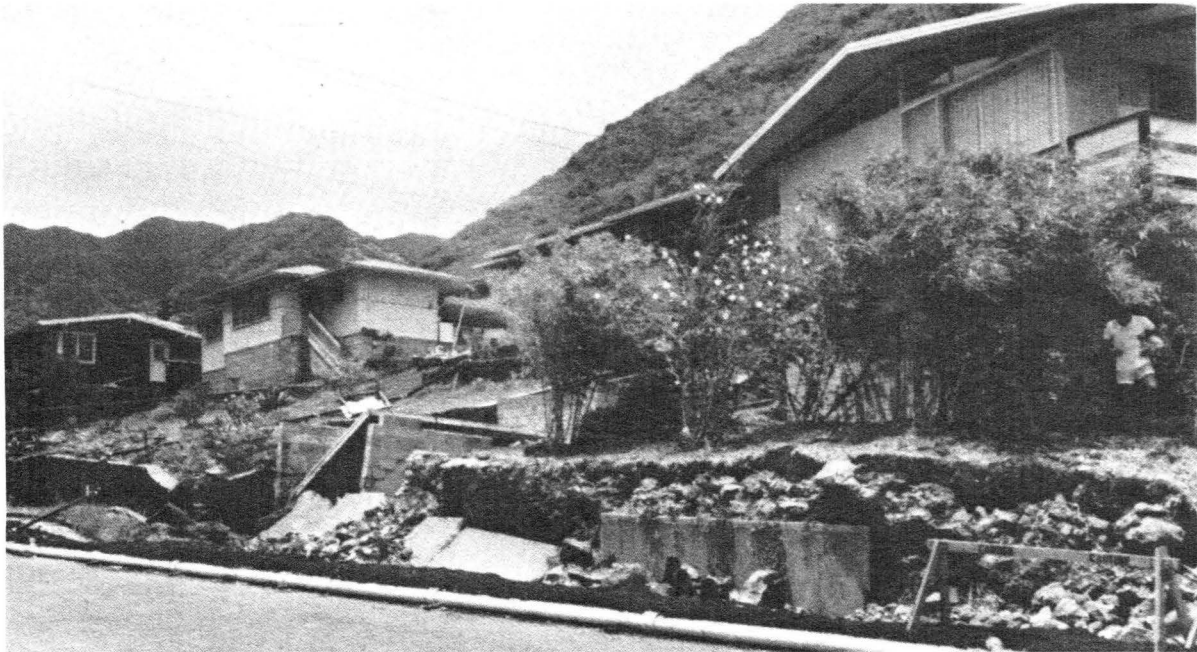
Vertisols are poor soils for engineering use, especially on steep areas. Slides in this area of Vertisols have damaged buildings and sidewalks.
