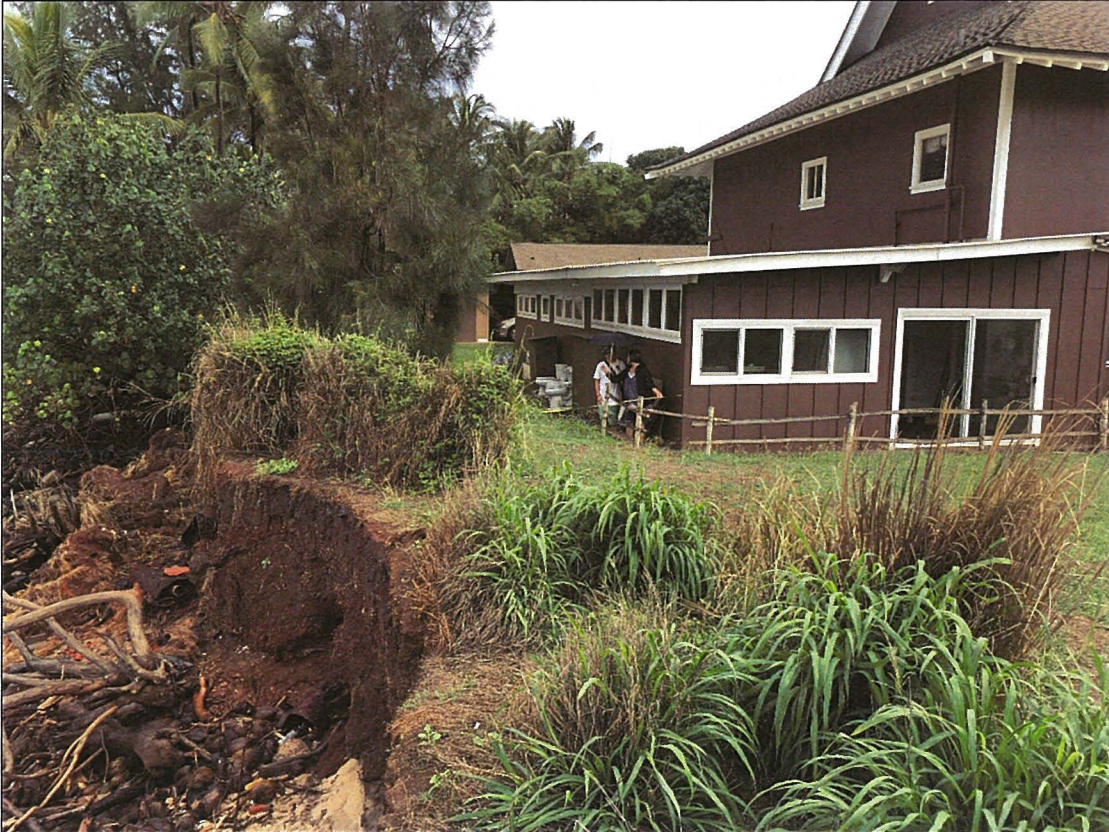
Erosion progression in proximity to the temple structure.
