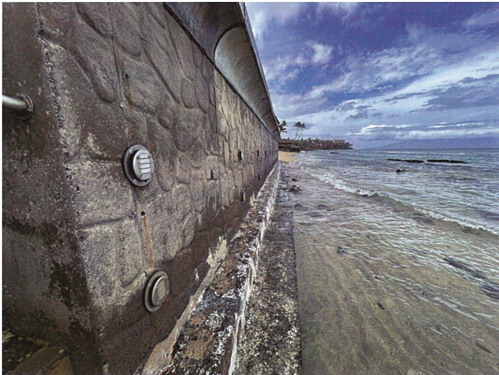
Southern section of seawall with sheet pile absent (04/20/22).
