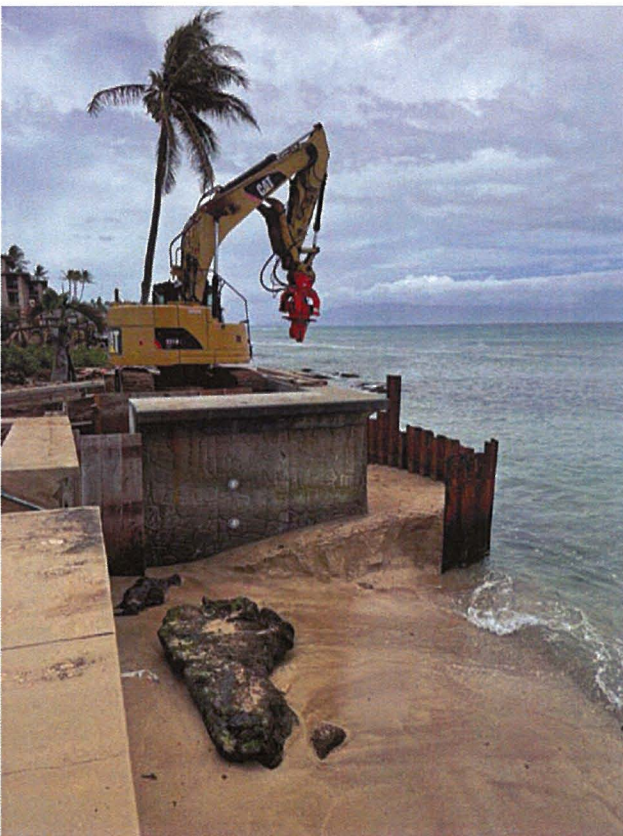
Northern portion of sheet pile removal in process (04/22/22).
