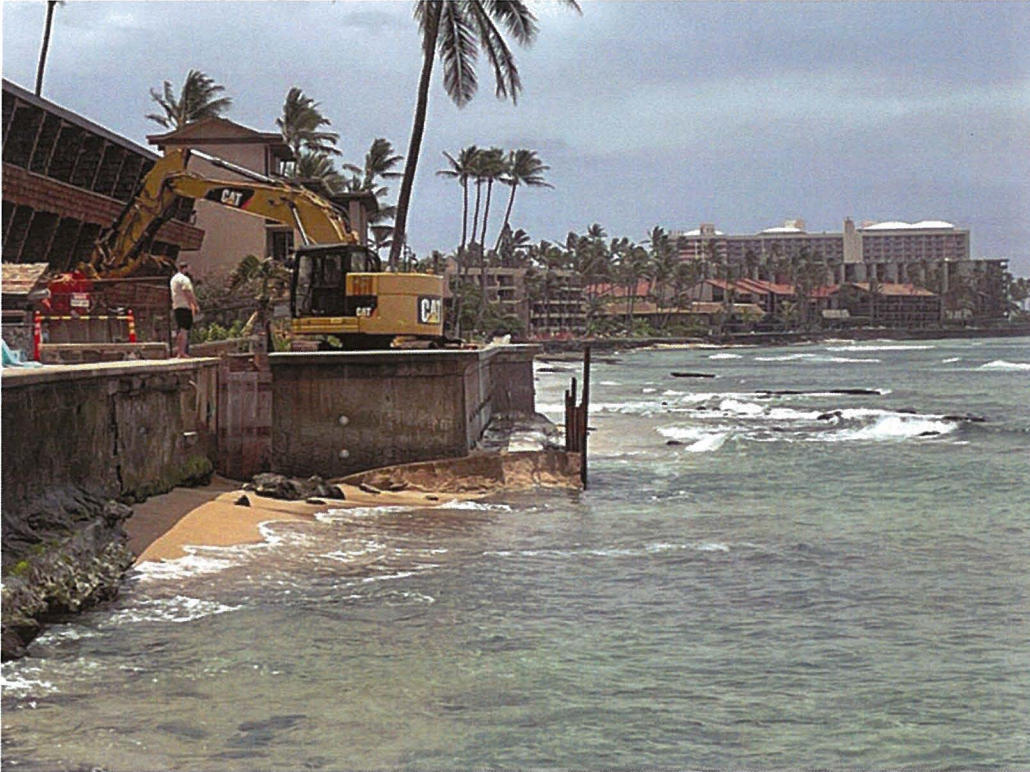
Northern portion of sheet pile removal in process (04/22/22).
