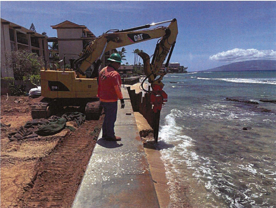
Facing south with removal of sheet pile in progress (04/20/22).
