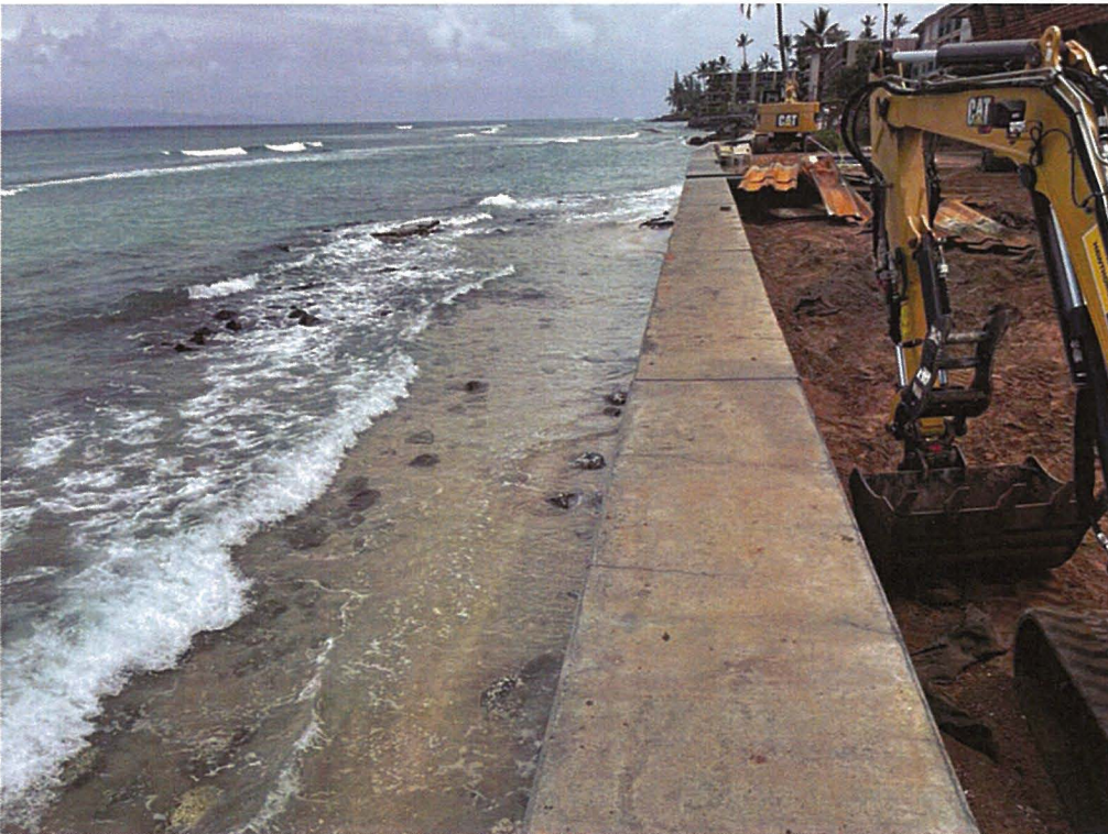
Northern portion of sheet pile removed (04/22/22).
