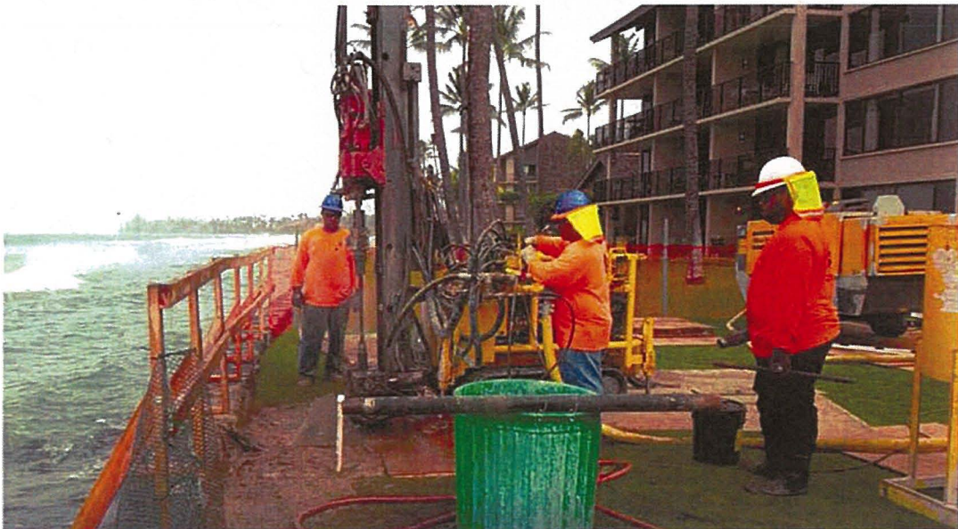
Figure 8 - County approved injection grouting to repair the seawall at the nearby Papakaea Condominium in 2015.
