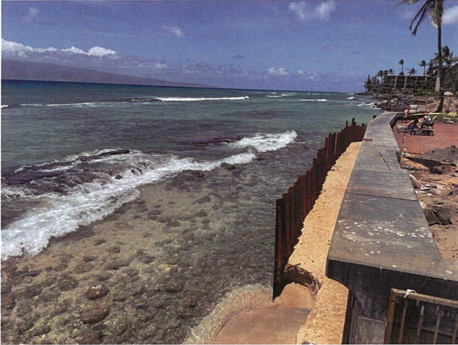
Northern portions of sheet pile present (04/20/22).
