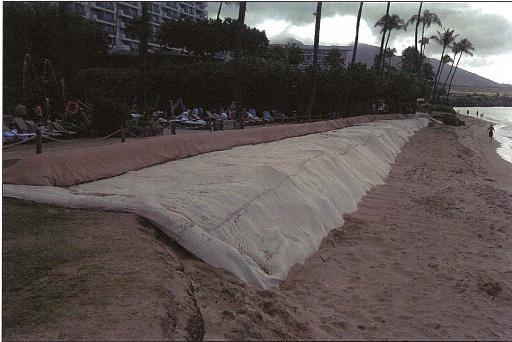
Figure 8. Phase 1 (2016) completed erosion skirt
