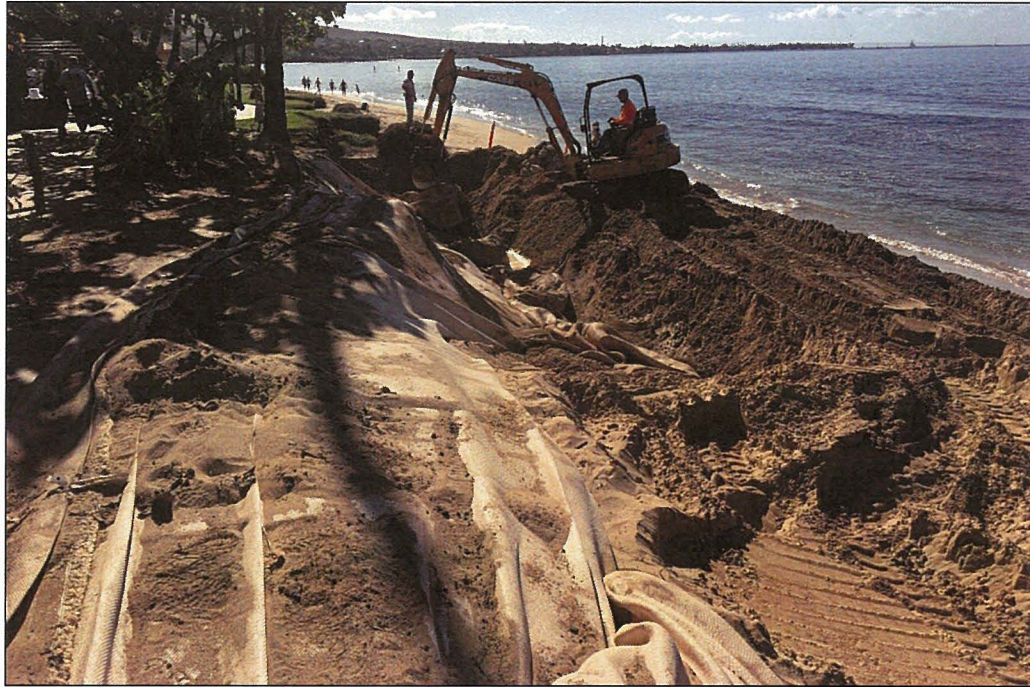
Figure 4. Removing existing erosion skirt (2016)
