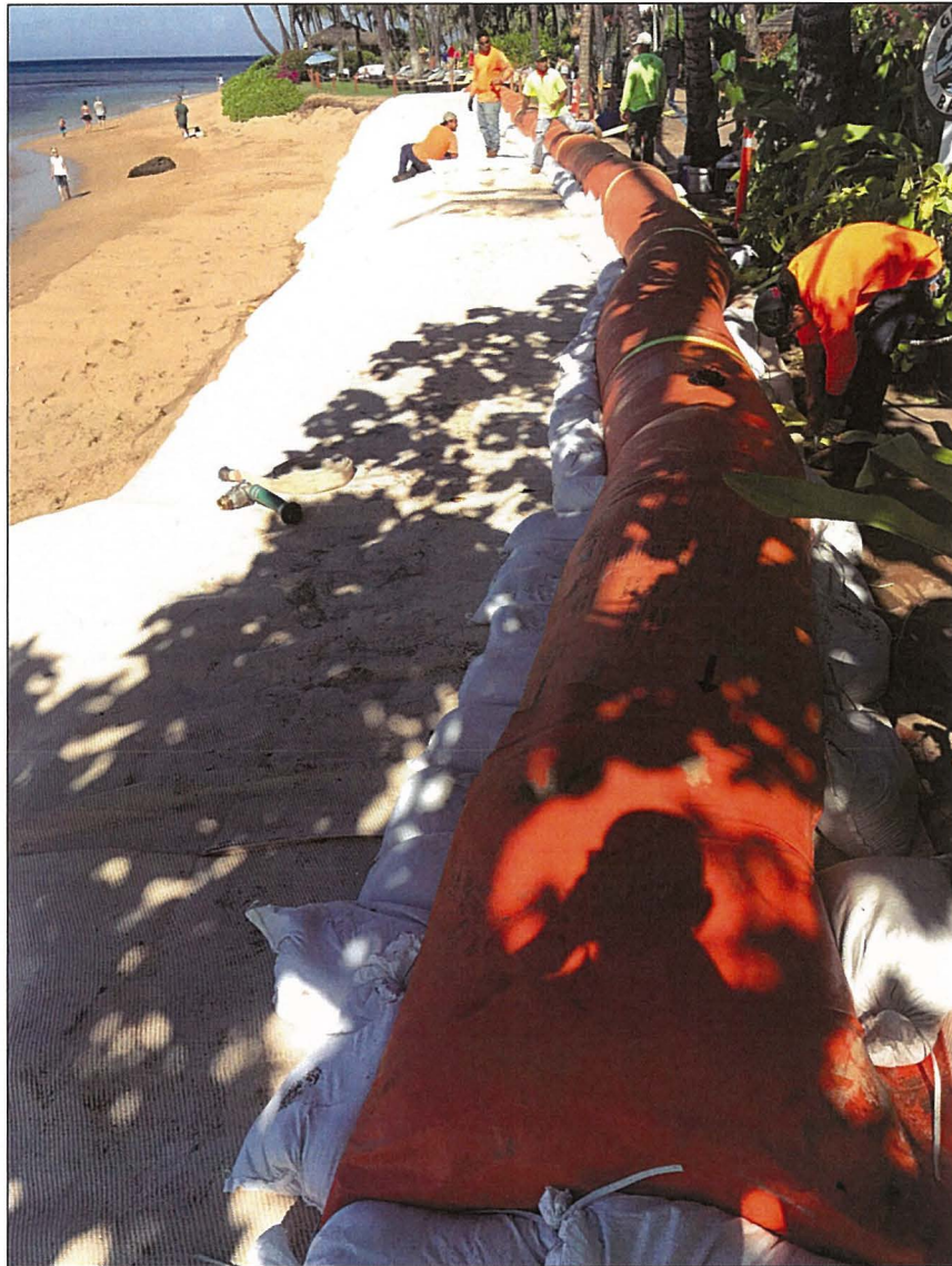
Figure 6. Tiger Dam, chock bags, and anchoring installation (2016)
