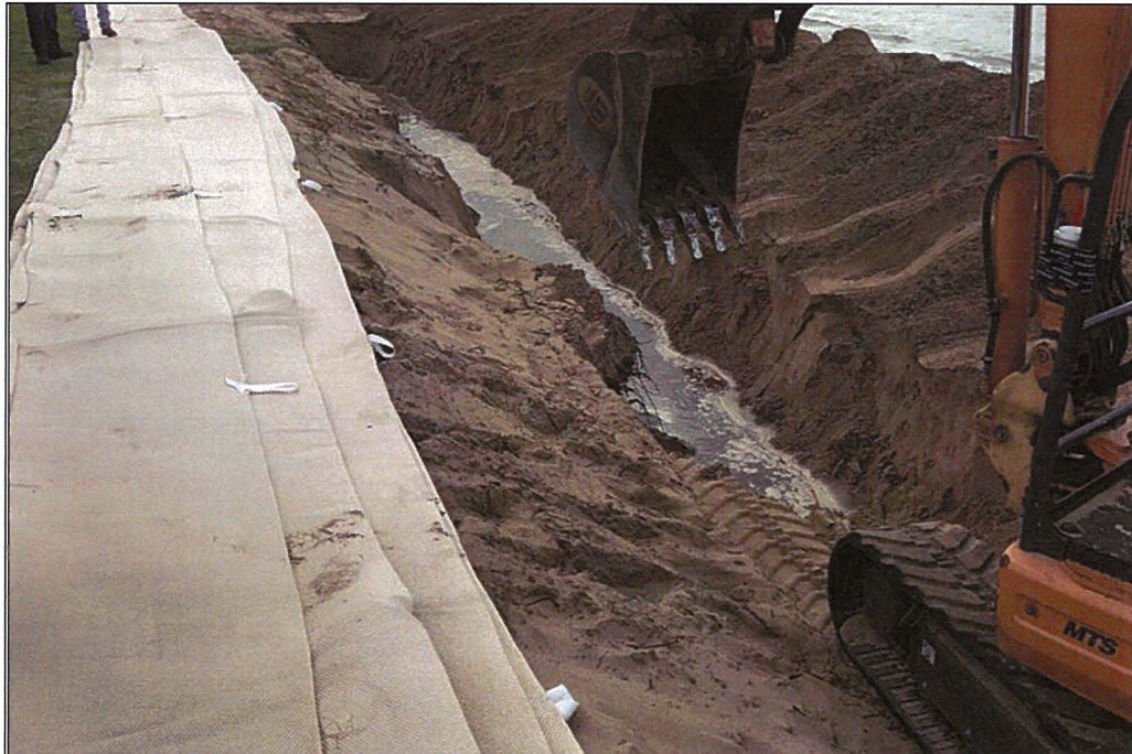
Figure 5. Digging the toe trench (2016)
