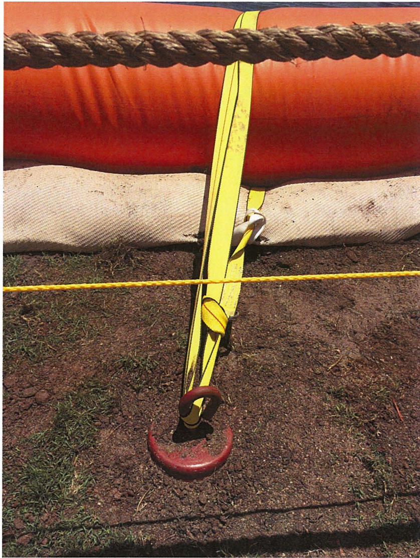
Figure 7. Tiger Dam and strongback anchoring (2016)
