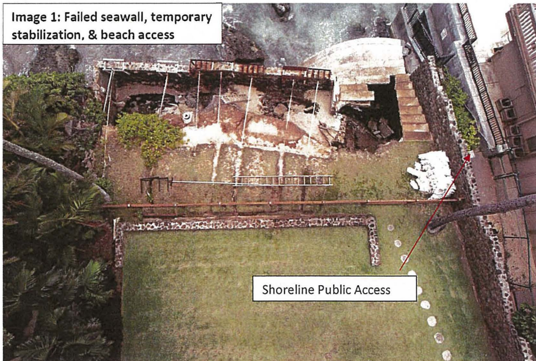
Image 2: Failed seawall and temporary stabilization.
