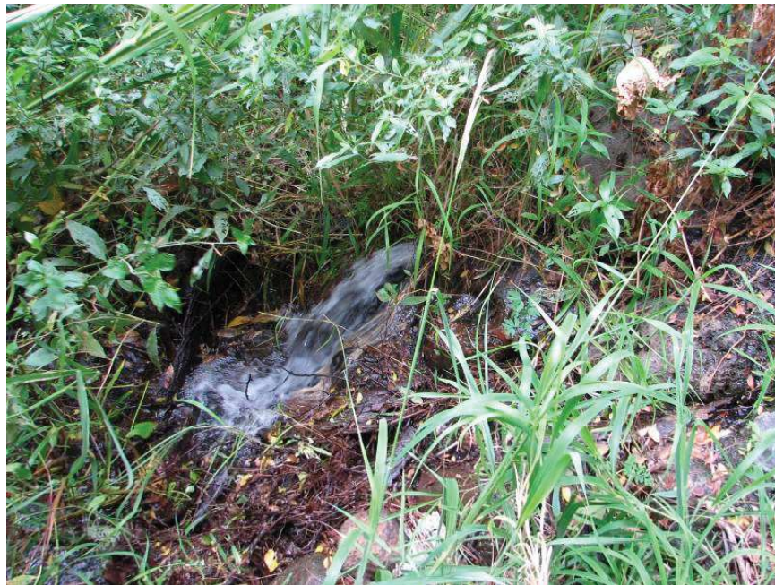
Figure 3. Seepage at the downstream face of Reservoir 3.
