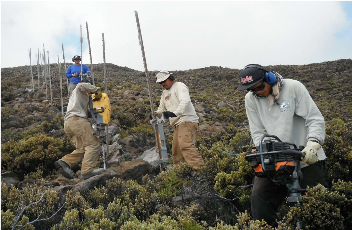
3 Fence crews building fence in the adjacent Nakula NAR in 2012. This fence was the first step towards ecosystem recovery.
