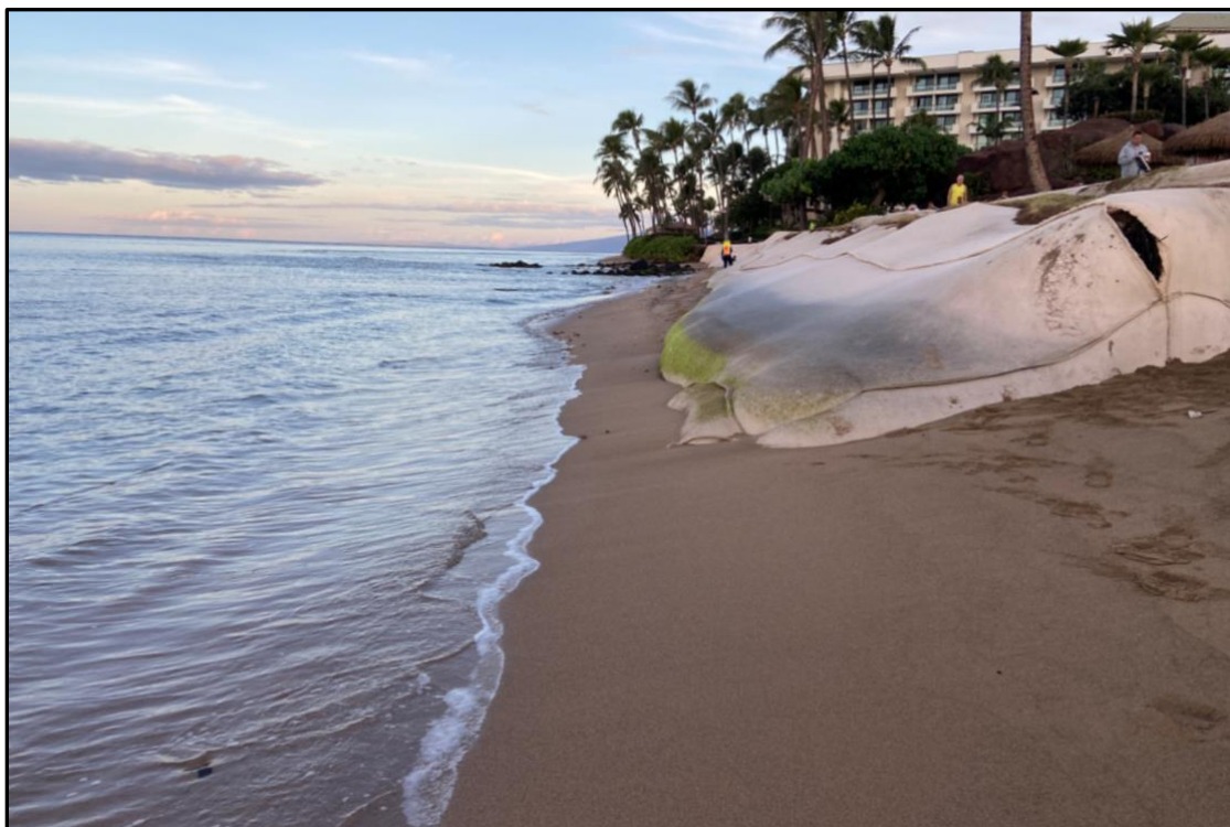
Photograph 2. Eastern end of the EEPS that still needs to be repaired. Photo date October 6, 2022, 6:33 am, tide level +0.2 ft mllw. Photo taken 16 minutes before lower low tide.
