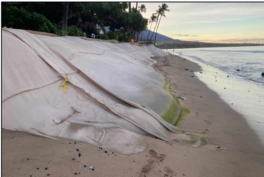
Photograph 1. Center of the EEPS that still needs to be repaired. Photo date October 6, 2022, 6:30 am, tide level +0.2 ft mllw. Photo taken 19 minutes before lower low tide.
