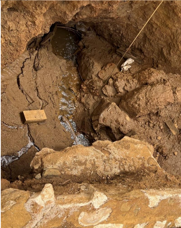
Figure 2 (above) shows the excavation around outlet intake and the lack of protection from internal erosion
