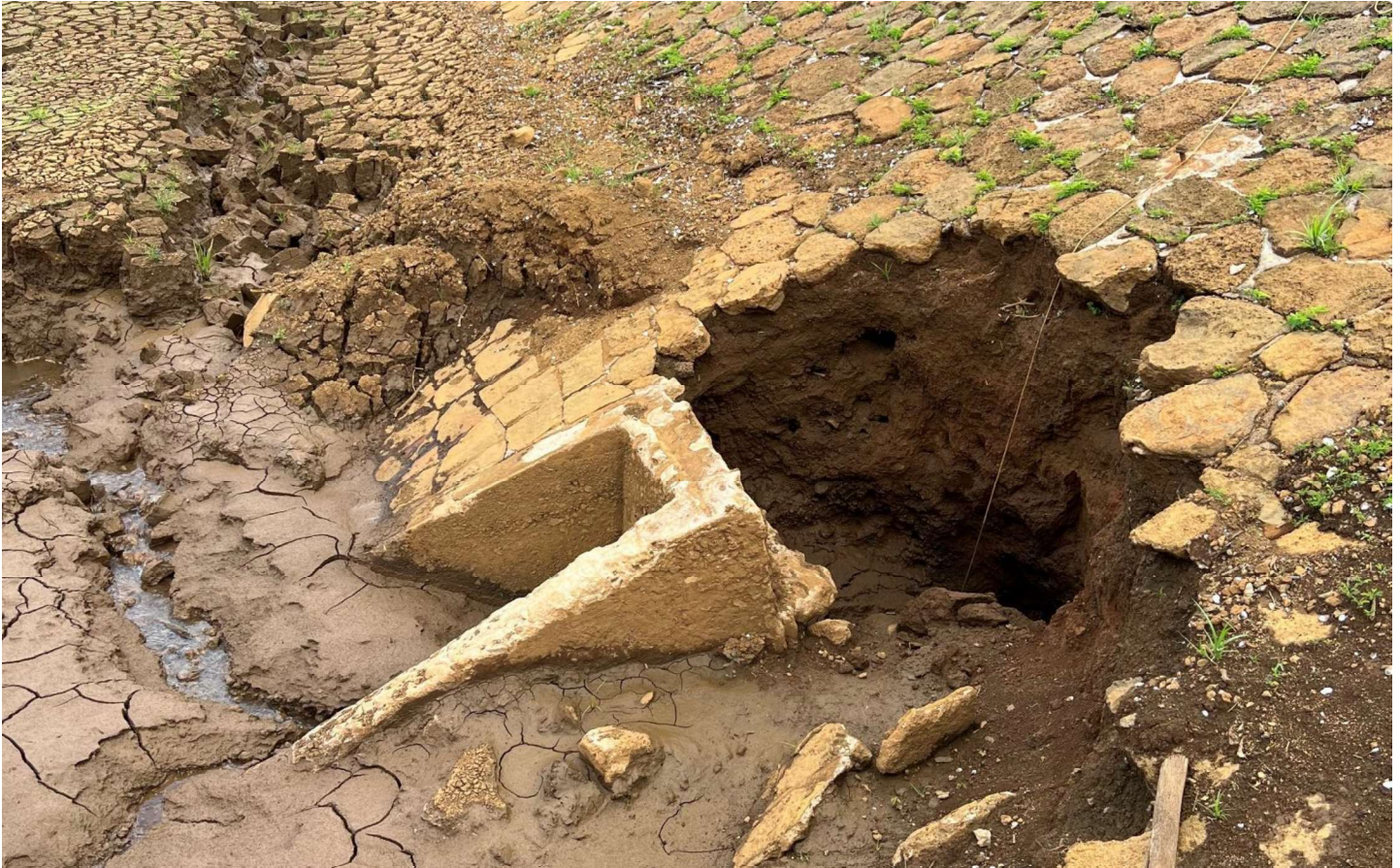
Figure 2 (above) shows the excavation around outlet intake and the lack of protection from internal erosion
