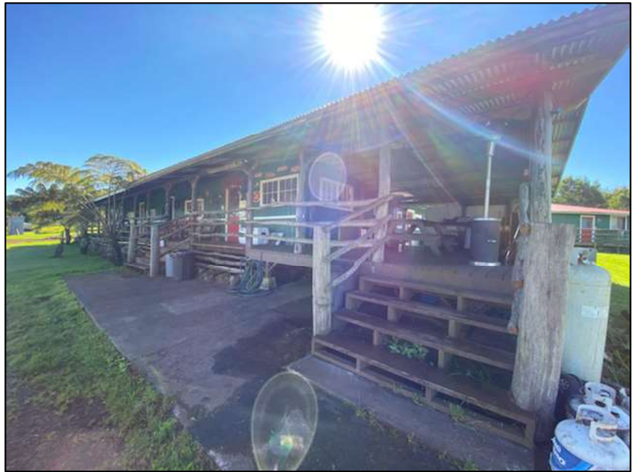
Figure 3. Main cabin at HA. Photo source: Forest Solutions, 2020.
