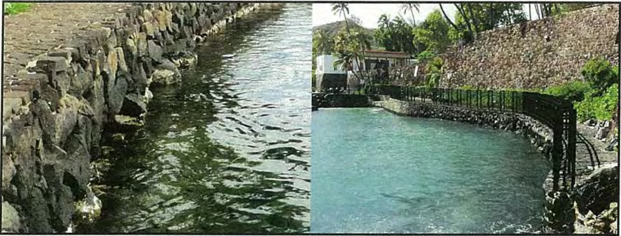
Note: Views of the seawall. TMK: (1) 3-1-041:seaward of 005.
