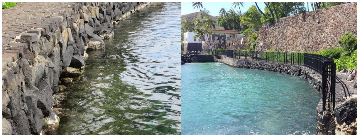
Figure 4: Detail of seawall and pedestrian walkway
