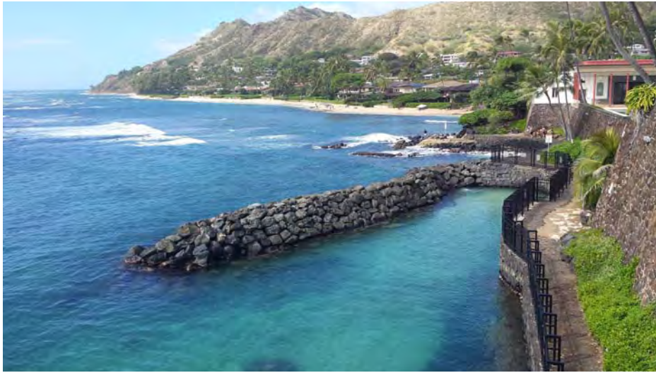
Current View of Diamond Head Breakwater from Balcony
