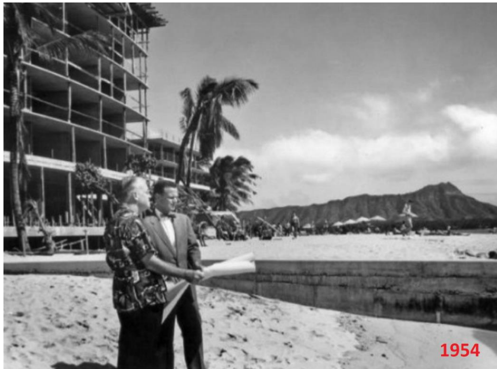
Outrigger Reef Waikiki Beach under construction 1954
