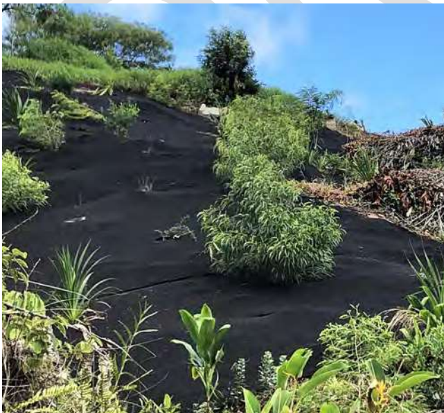
Figure 21. Weed mat suppressing weeds. Kaneohe, O'ahu.
