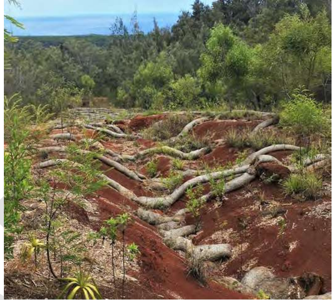
Figure 27: Coconut coir logs used to capture eroding soil. Waimea, O'ahu.
