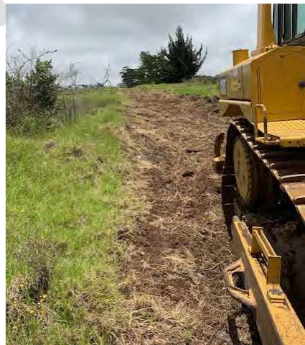
Figure 22. Fuelbreak being installed with a dozer. North Kona, Hawai'i.
