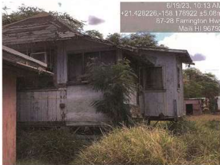
Figure 2: Middle structure (2nd house)
