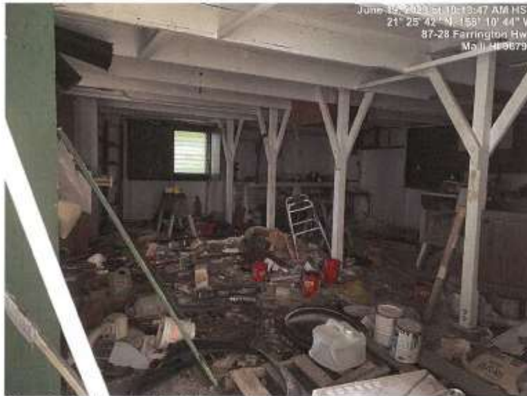
Figure 3: Interior of workshop between the two houses
