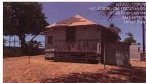
Tenant intends to demolish House 2
