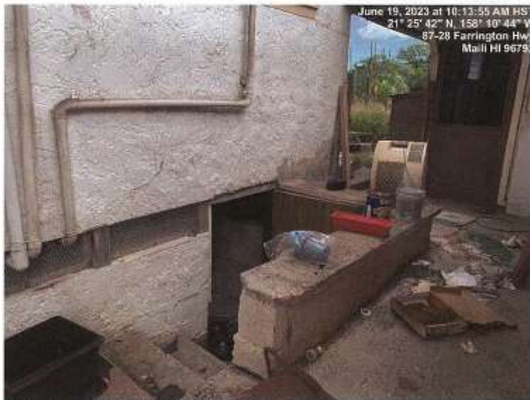
Figure 4: Access to beneath front house
