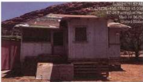
House 2 is not being used.
