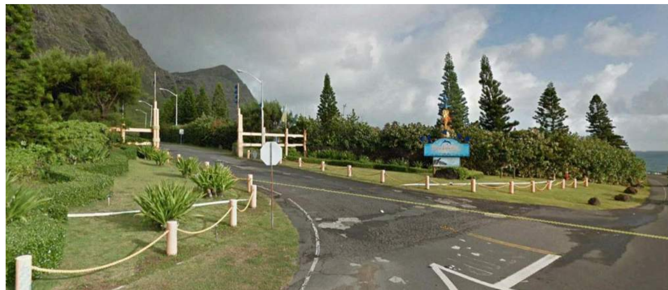
Existing Conditions - looking north
