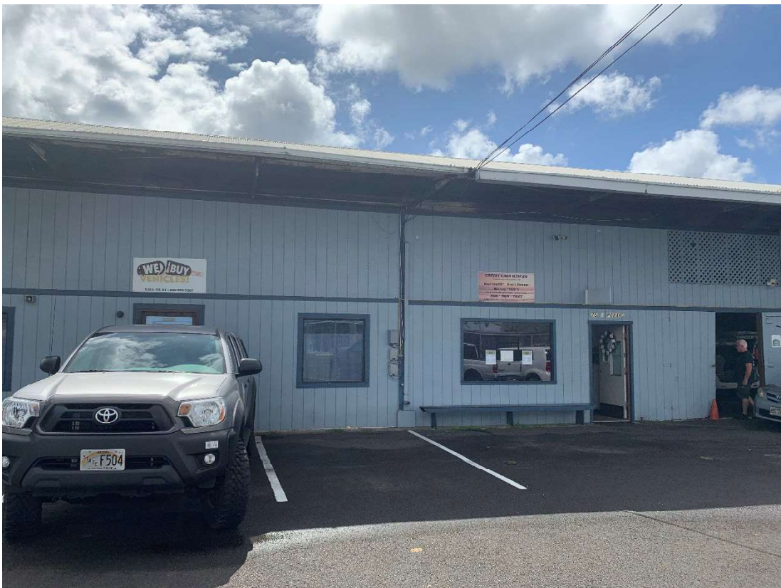
FRONT OF WAREHOUSE
