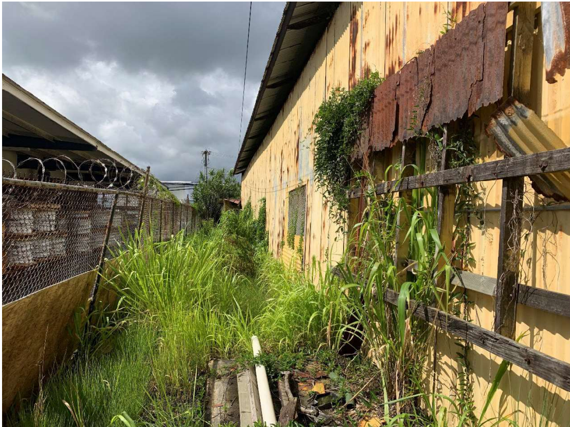
REAR VIEW OF WAREHOUSE
