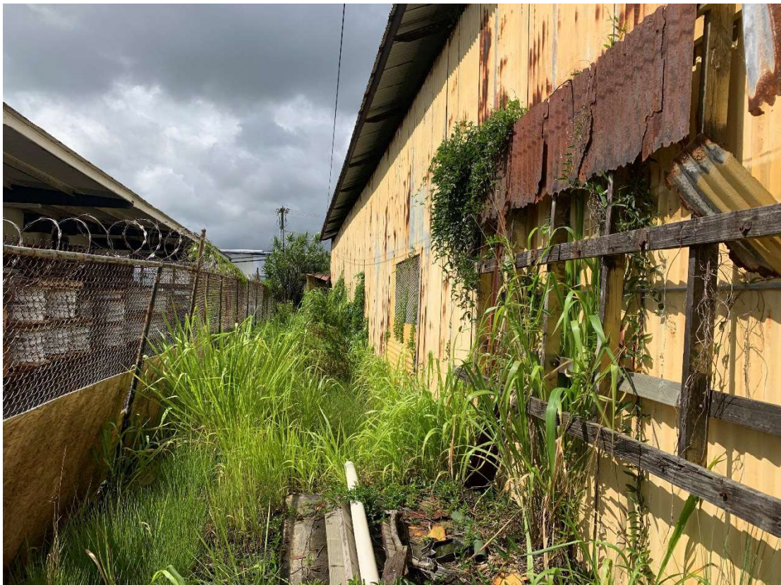
REAR VIEW OF WAREHOUSE
