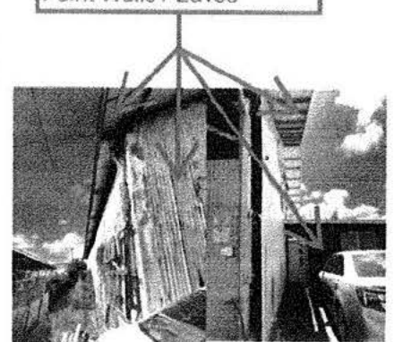
Paint Walls / Eaves
