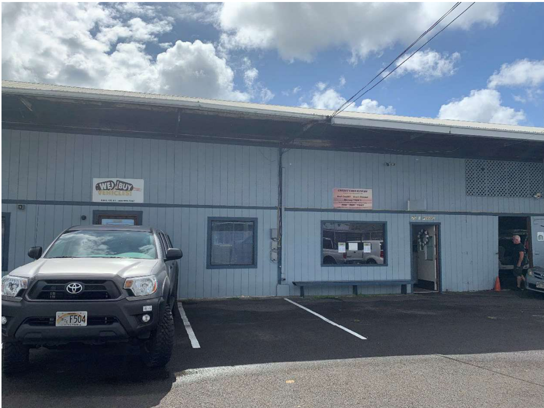
FRONT OF WAREHOUSE
