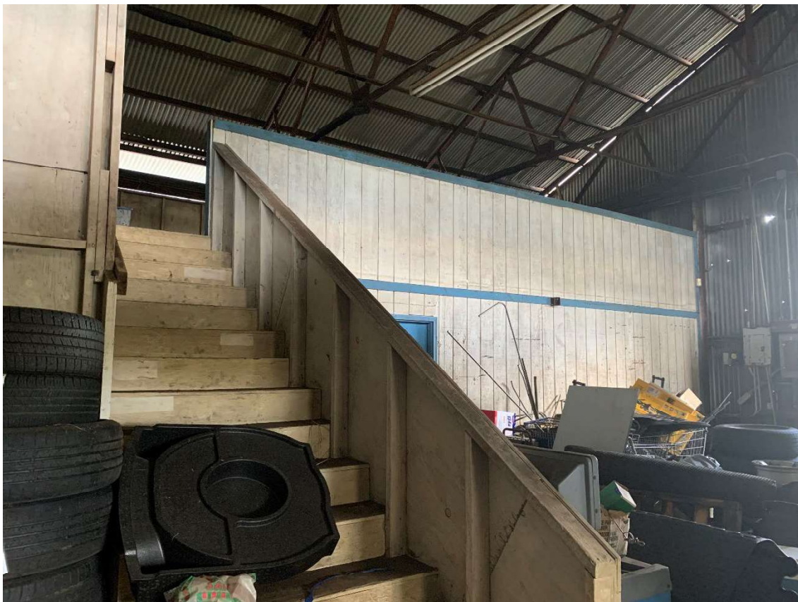
STAIRWAY TO LOFT STORAGE AREA
