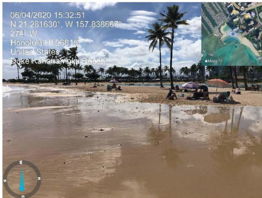
Figure 3. Photographs of backshore flooding resulting from high tides and south swell (photo date June 4, 2020). This condition is most severe during summer King tides and can be expected to worsen with increasing sea levels.
