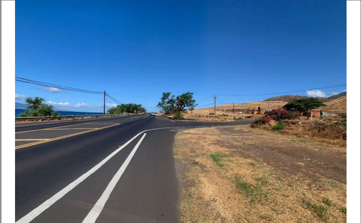
Ingress / Egress Includes Existing Left Turn Storage Lane Heading South from Lahaina (Photo 1)
