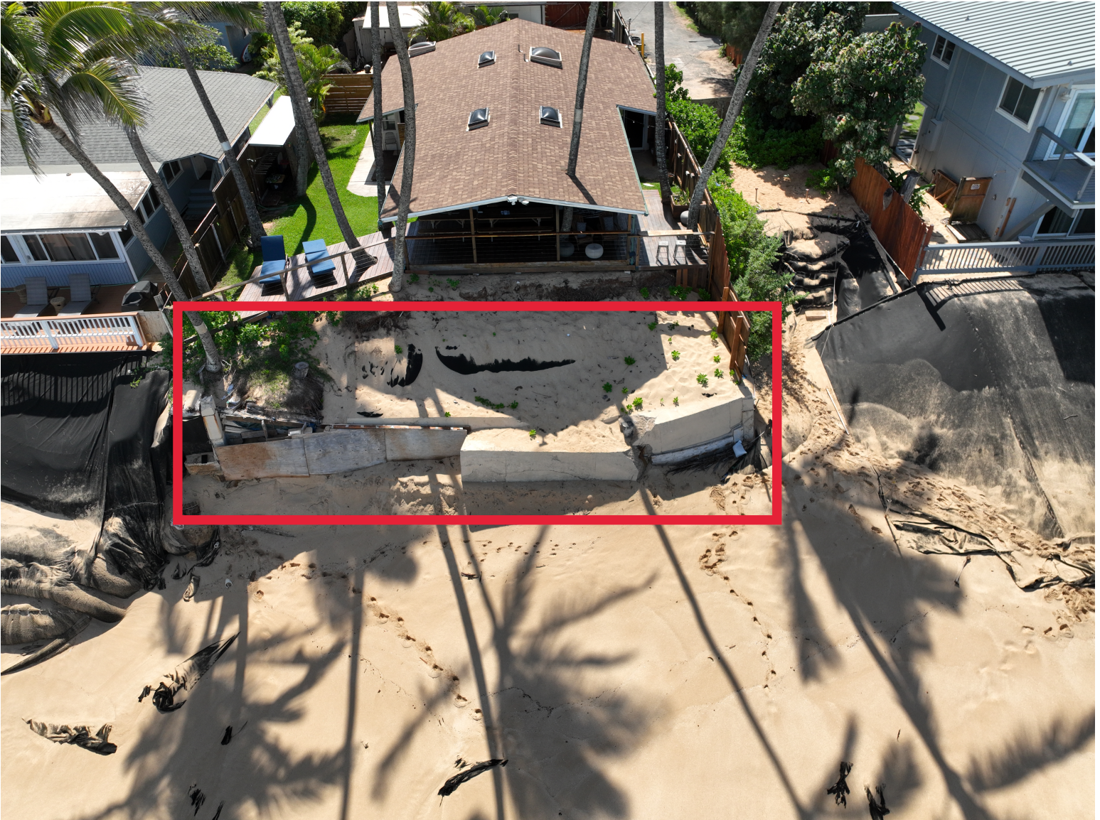
10/2/2023 OCCL Photo Showing Approximate Area of Proposed Temporary Erosion Control Structure in the Shoreline Area Fronting the Subject Parcel
