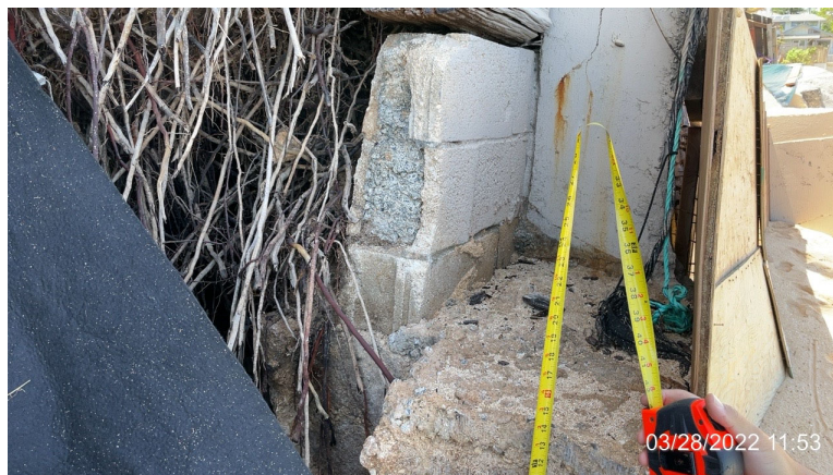
Photo 17: North corner of seawall (original materials investigation), zoomed with measurement
