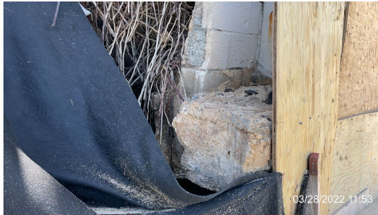
Photo 16: North corner of seawall (original materials investigation), zoomed
