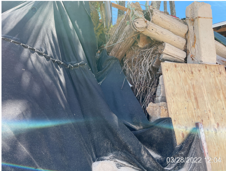
Photo 14: North corner of seawall (original materials investigation)
