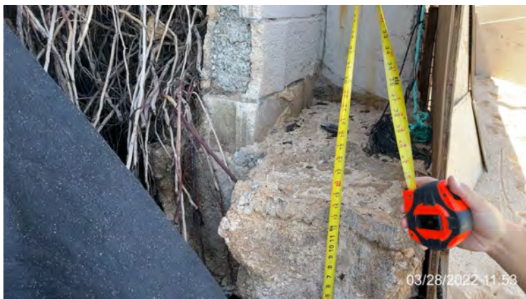
Photo 18: North corner of seawall (original materials investigation), zoomed with measurement
