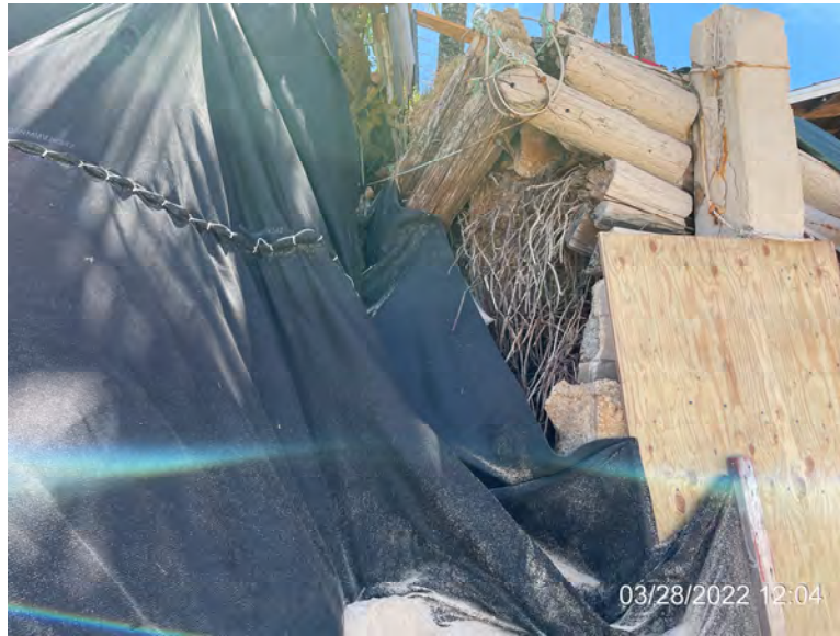
Photo 14: North corner of seawall (original materials investigation)
