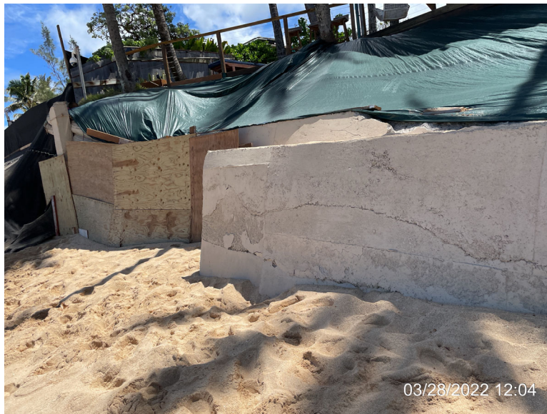
Photo 6: North side of property seawall (about mid-way) facing mauka
