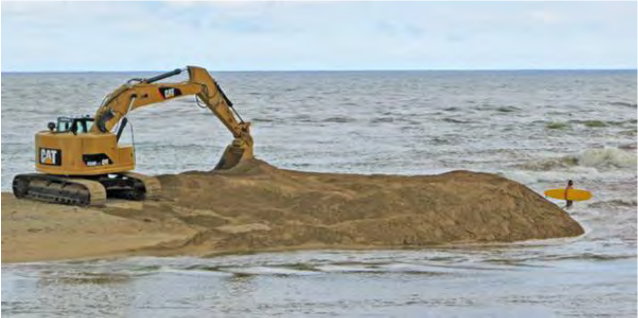
Excavator on beach at Kauai for Wailua River Mouth clearing
