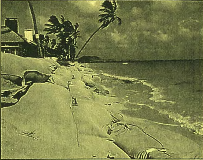
Geotextile bags in the form of a soft revetment.
