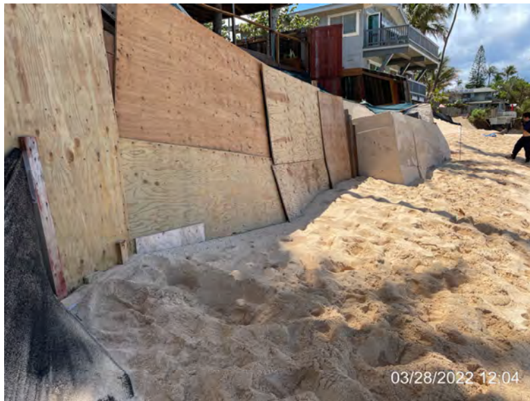
Photo 8: Length of property seawall taken from North facing South
