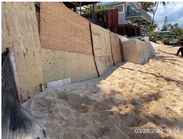
Photo 8: Length of property seawall taken from North facing South
