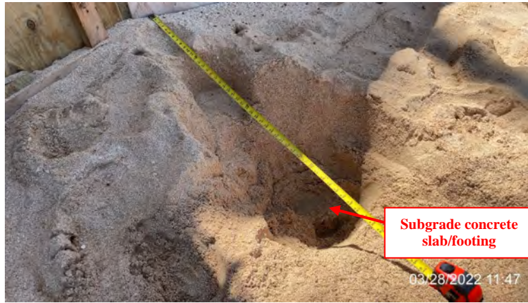
Photo 11: Probing North end of seawall for depth of footings and structures.
