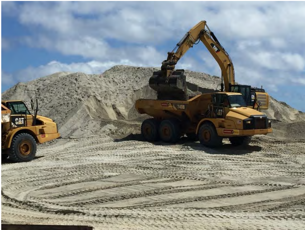
Excavator and Trucks on Waikiki Beach 2021
