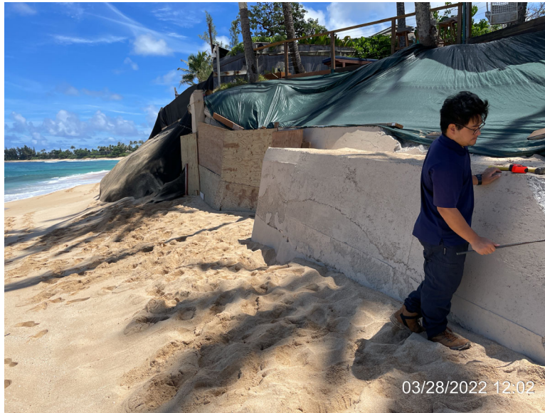
Photo 5: North side of property seawall (about mid-way) facing North
