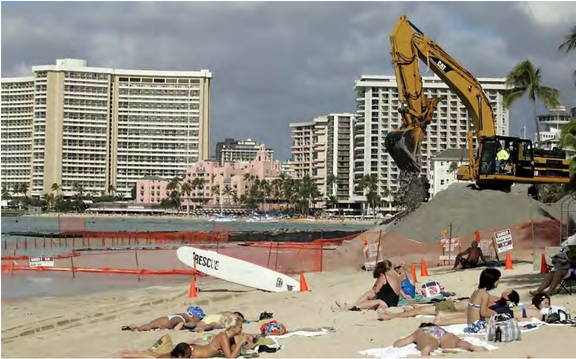
Excavator on Waikiki Beach (Kuhio Beach Sand Replenishment Demonstration) 2006
