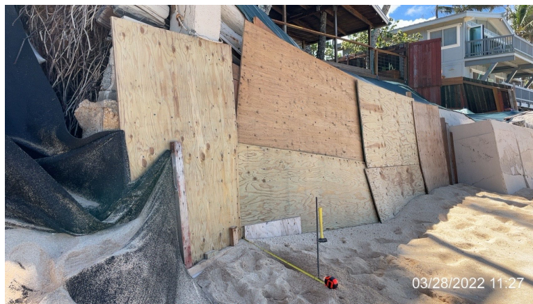
Photo 10: Probing North end of seawall for depth of footings and structures.
