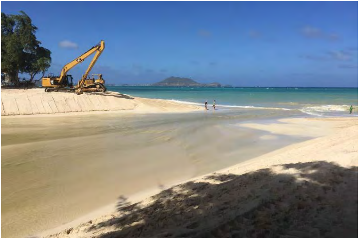
Excavator and Bulldozer clearing Kaelepulu Stream at Kailua Beach Park
