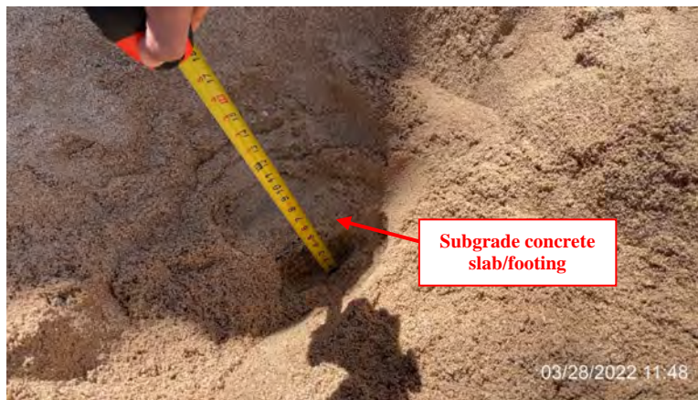
Photo 12: Probing North end of seawall for depth of footings and structures.
