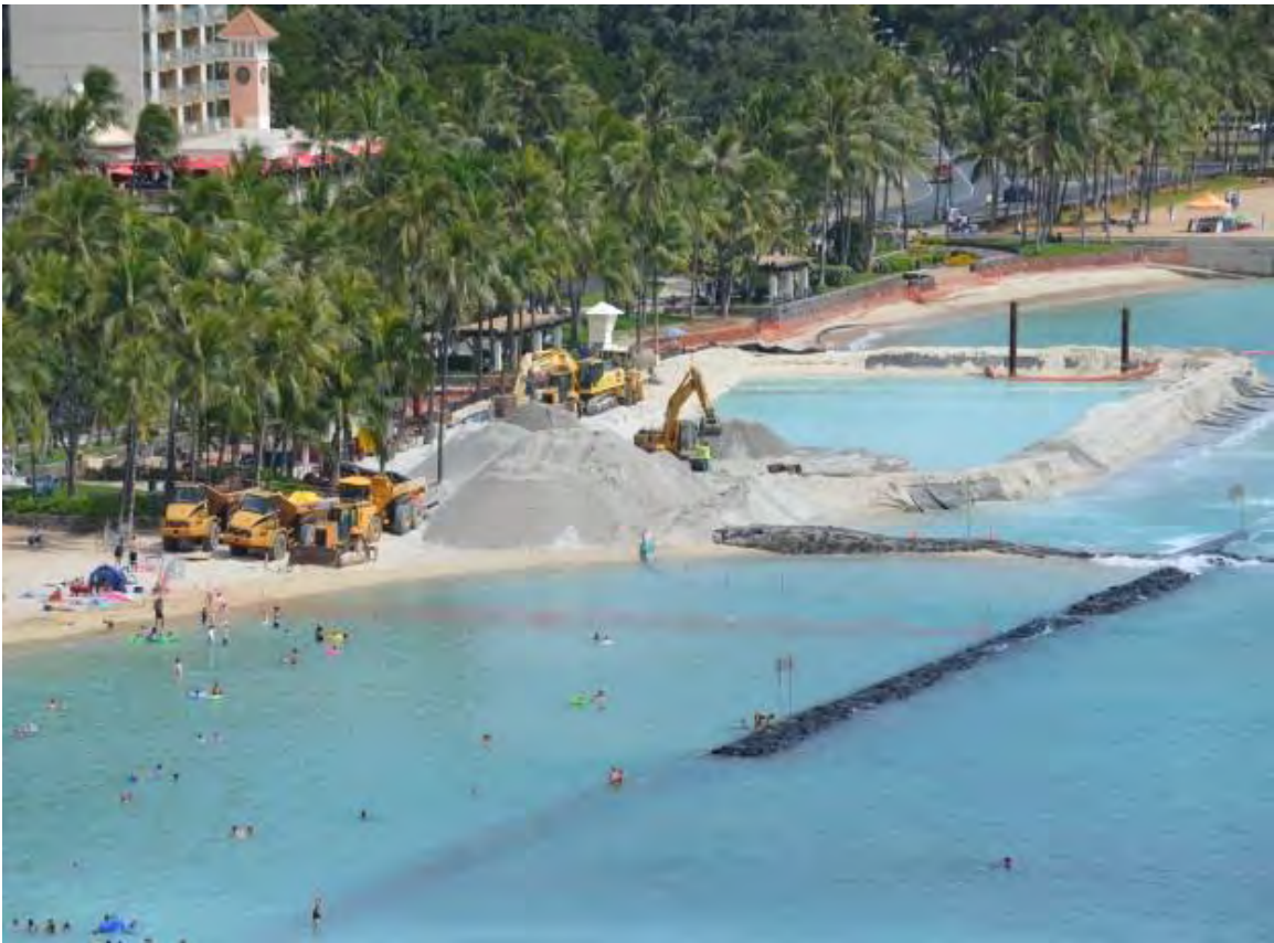
Excavator and Trucks on Waikiki Beach (2012)
