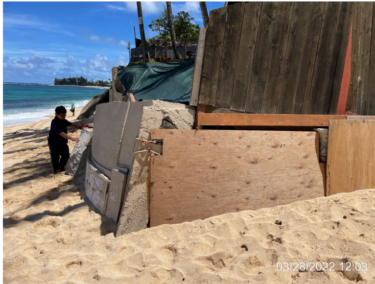
Photo 1: South corner of property seawall facing North
