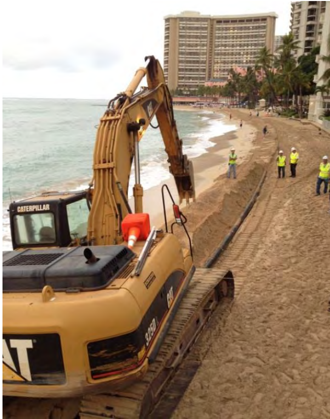
Excavator on Waikiki Beach (2012)
