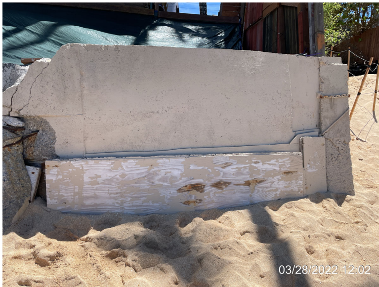
Photo 2: South corner of property seawall facing mauka
