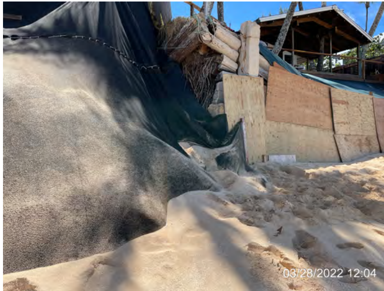
Photo 9: North corner of seawall facing Mauka
