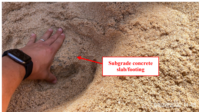
Photo 13: Probing North end of seawall for depth of footings and structures.
