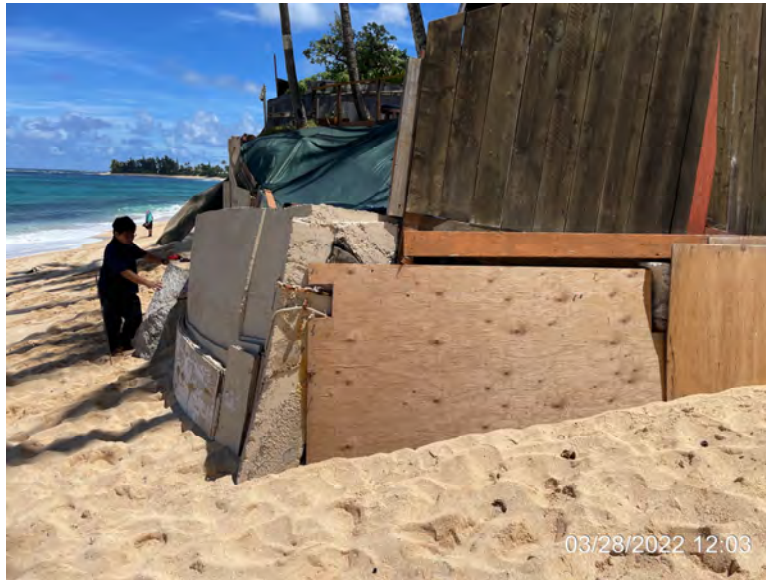
Photo 1: South corner of property seawall facing North
