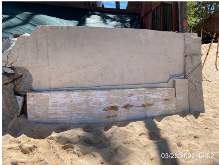
Photo 2: South corner of property seawall facing mauka
