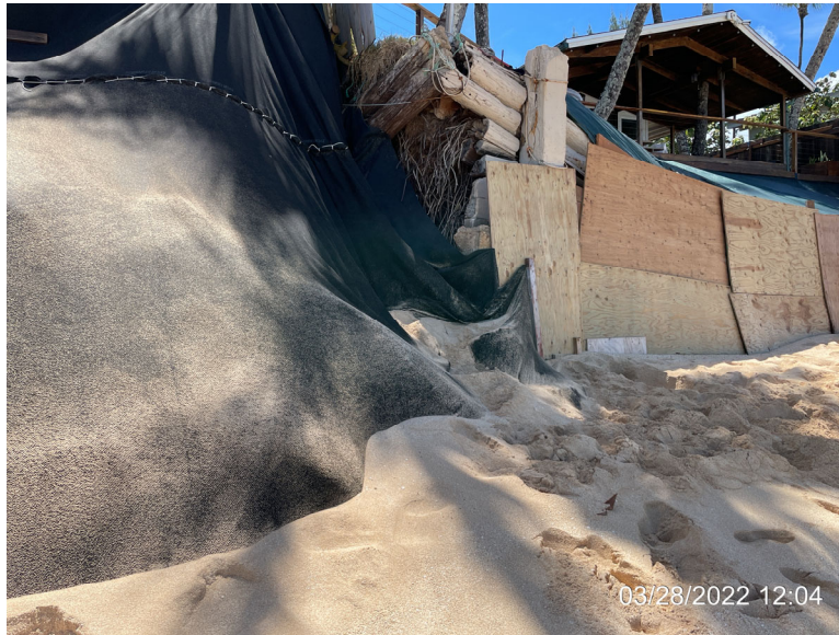
Photo 9: North corner of seawall facing Mauka
