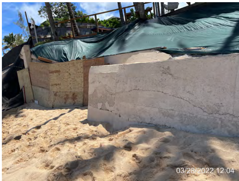
Photo 6: North side of property seawall (about mid-way) facing mauka
