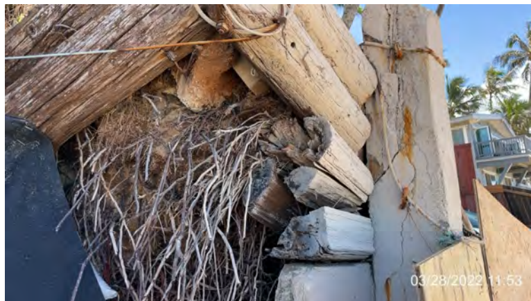
Photo 15: North corner of seawall (original materials investigation), zoomed
