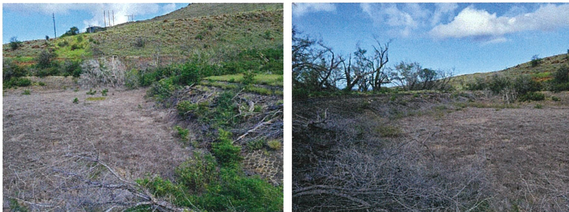
Figure 2. Ukumehame Reservoirs No. 2 (left) and No. 3 (right). (2021)
